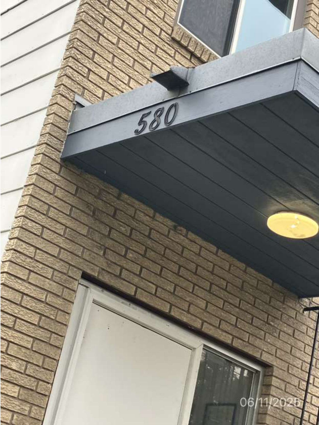
580 Minnehaha Ave E.Photos before and After done by Crew 6-11-25
