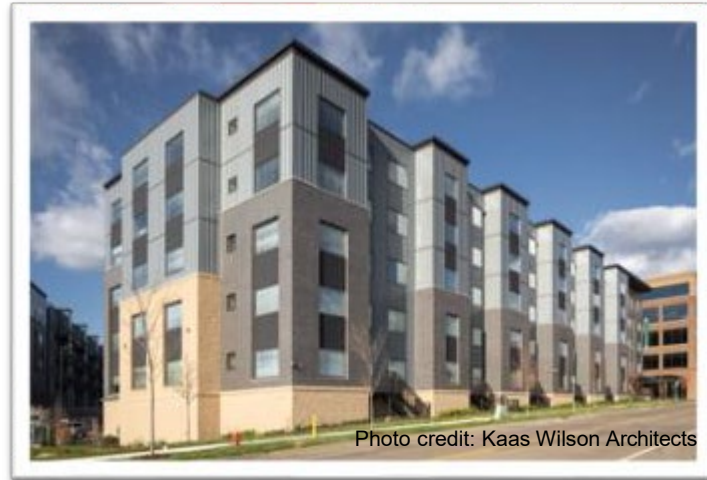
West Side Flats, Verdant Apartments. Completed 2021 Second multifamily building in Minnesota to achieve Passive House Institute US Certification
