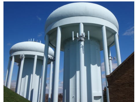
Highland Water Tower
