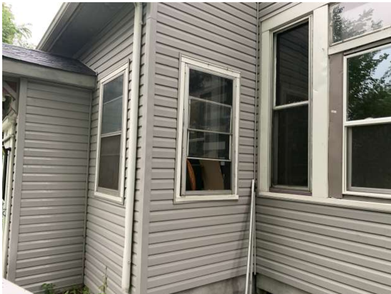
342 Bates Ave.photos from CE
