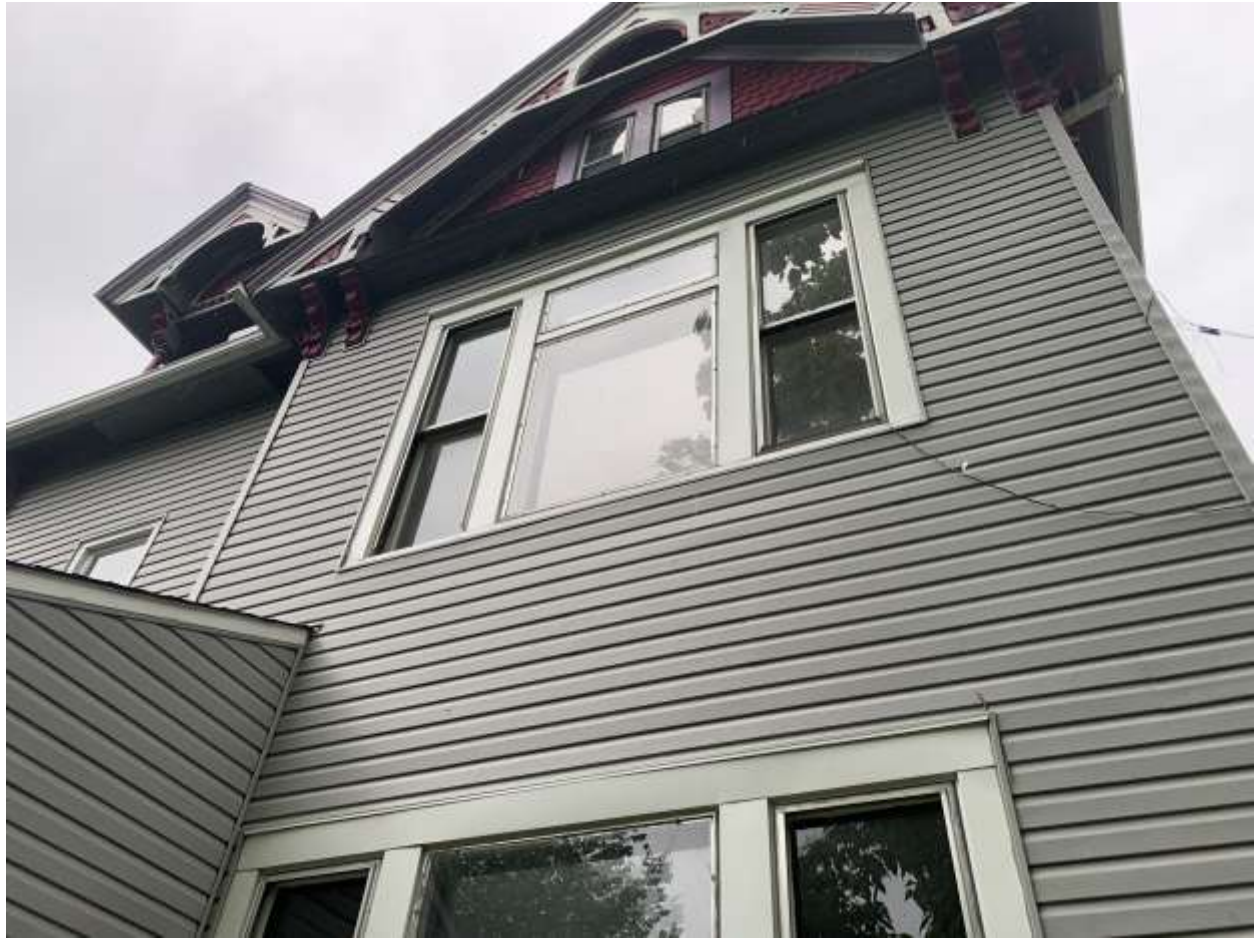
342 Bates Ave.photos from CE
