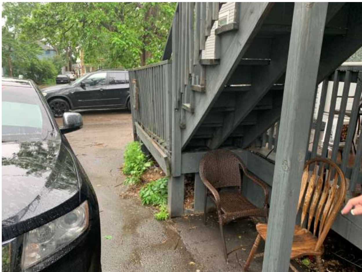
342 Bates Ave.photos from CE
