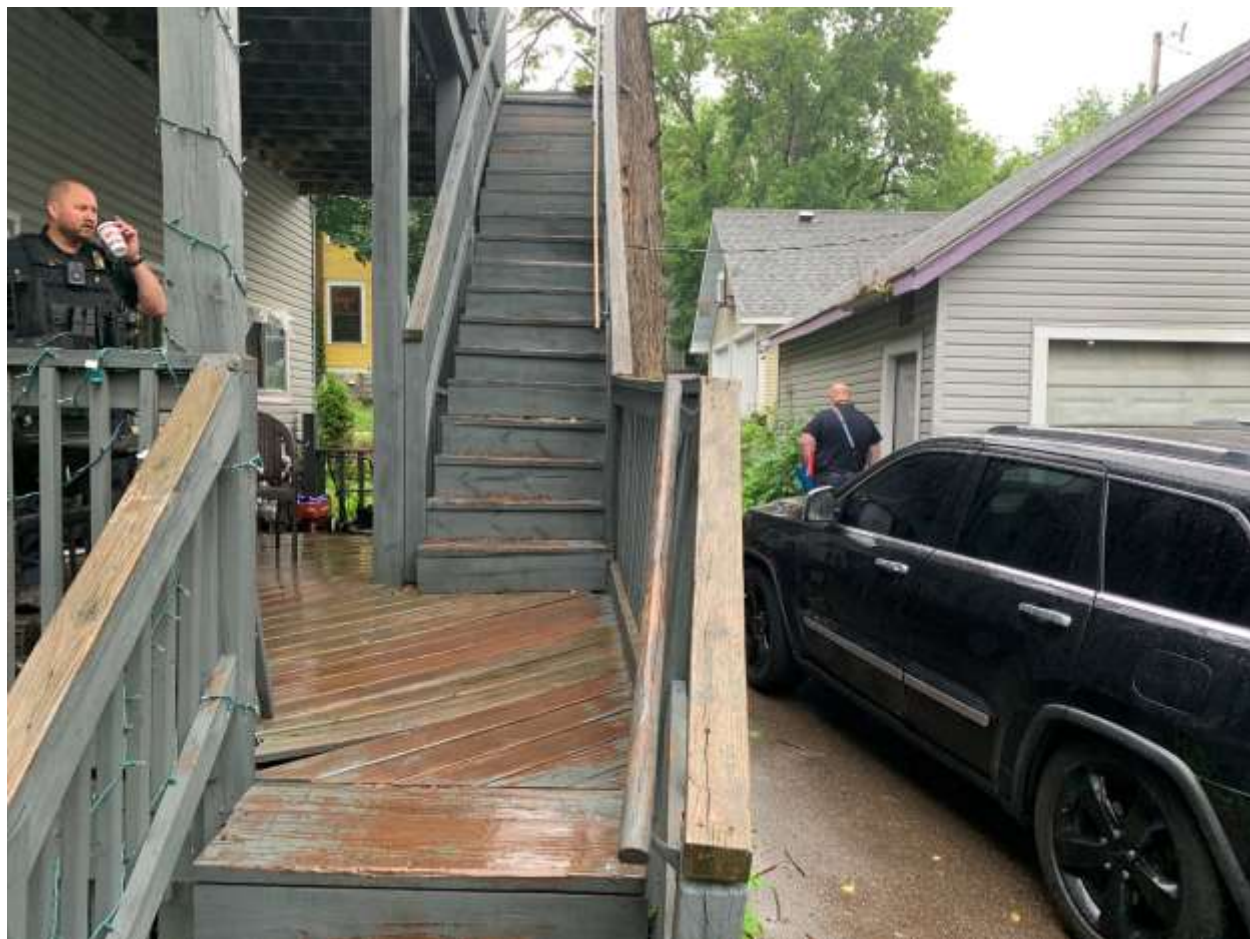
342 Bates Ave.photos from CE
