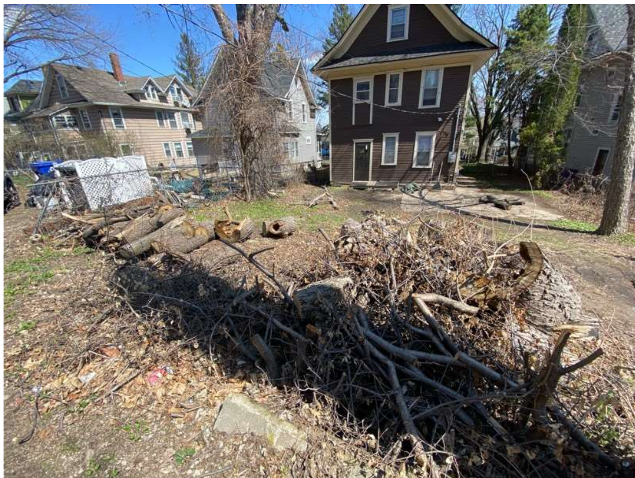
1119 Edgerton St. Photo from SA Order 4-22-25
