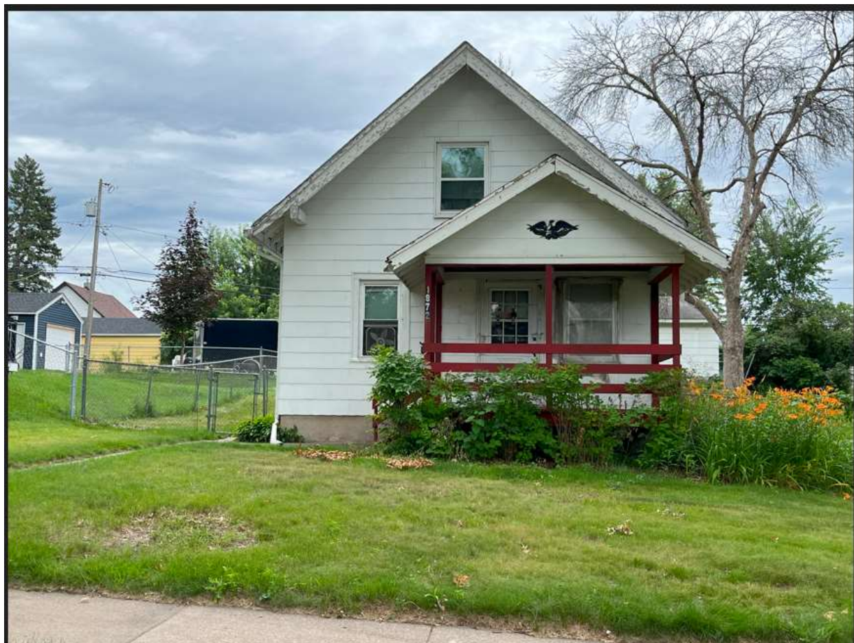
1872 Clear Ave photos 7-22-25
