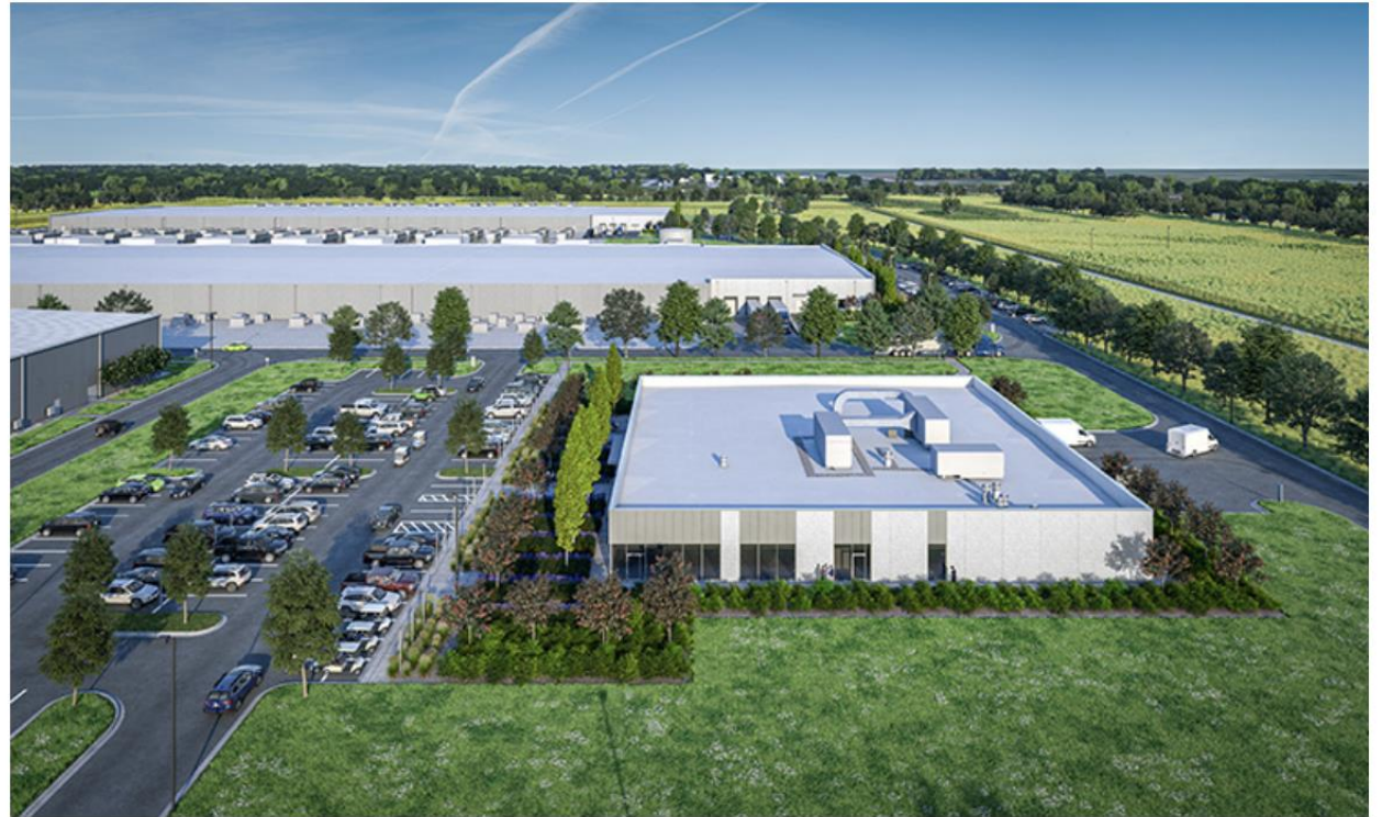
Rendering of Meta's new 715,000-square-foot data center in Rosemount PHOTO COURTESY OF META PLATFORMS INC.
