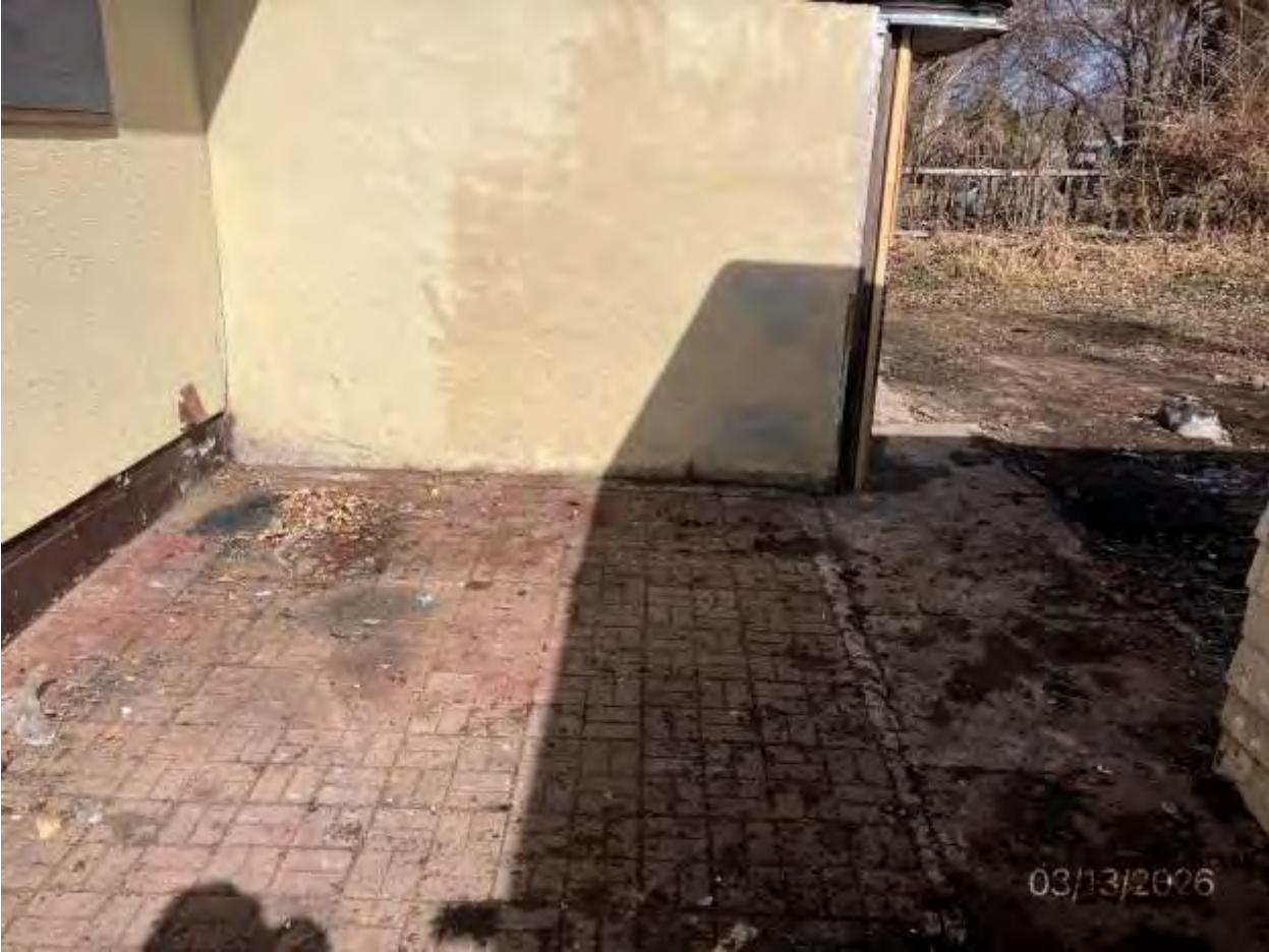
1164-1166 Cumberland St. Photos Before/After Clean Up 3-30-26
