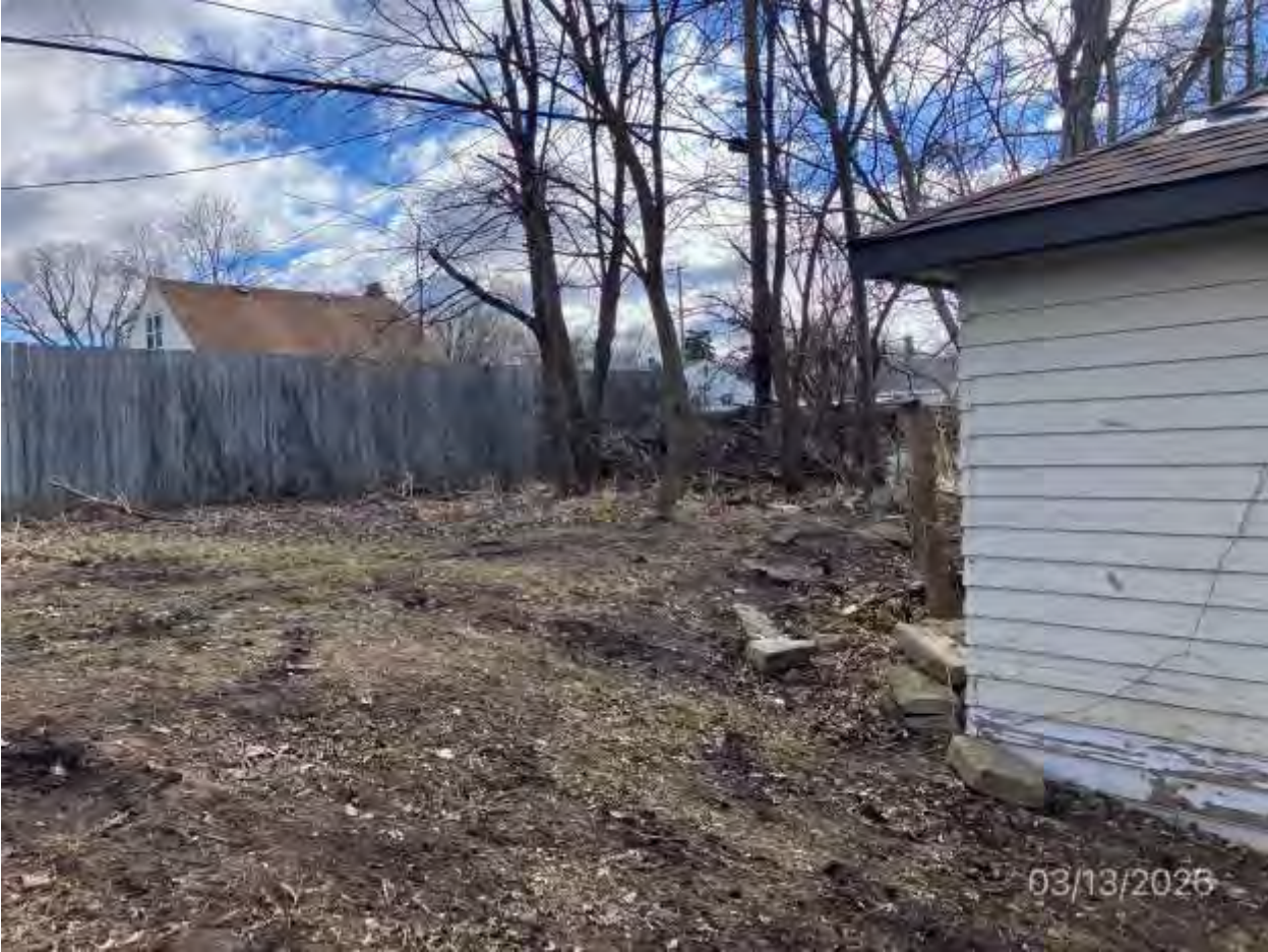
1164-1166 Cumberland St. Photos Before/After Clean Up 3-30-26
