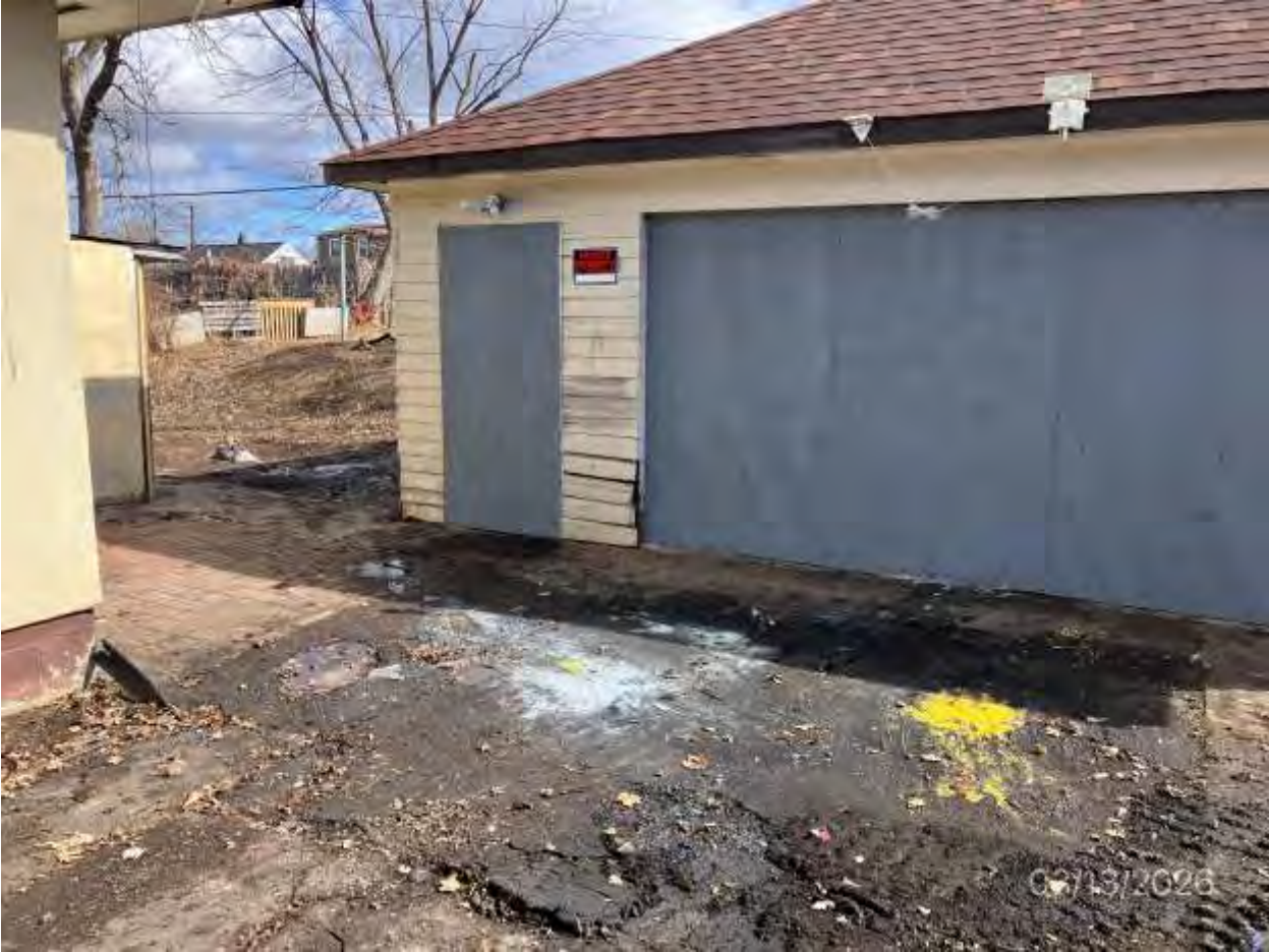
1164-1166 Cumberland St. Photos Before/After Clean Up 3-30-26
