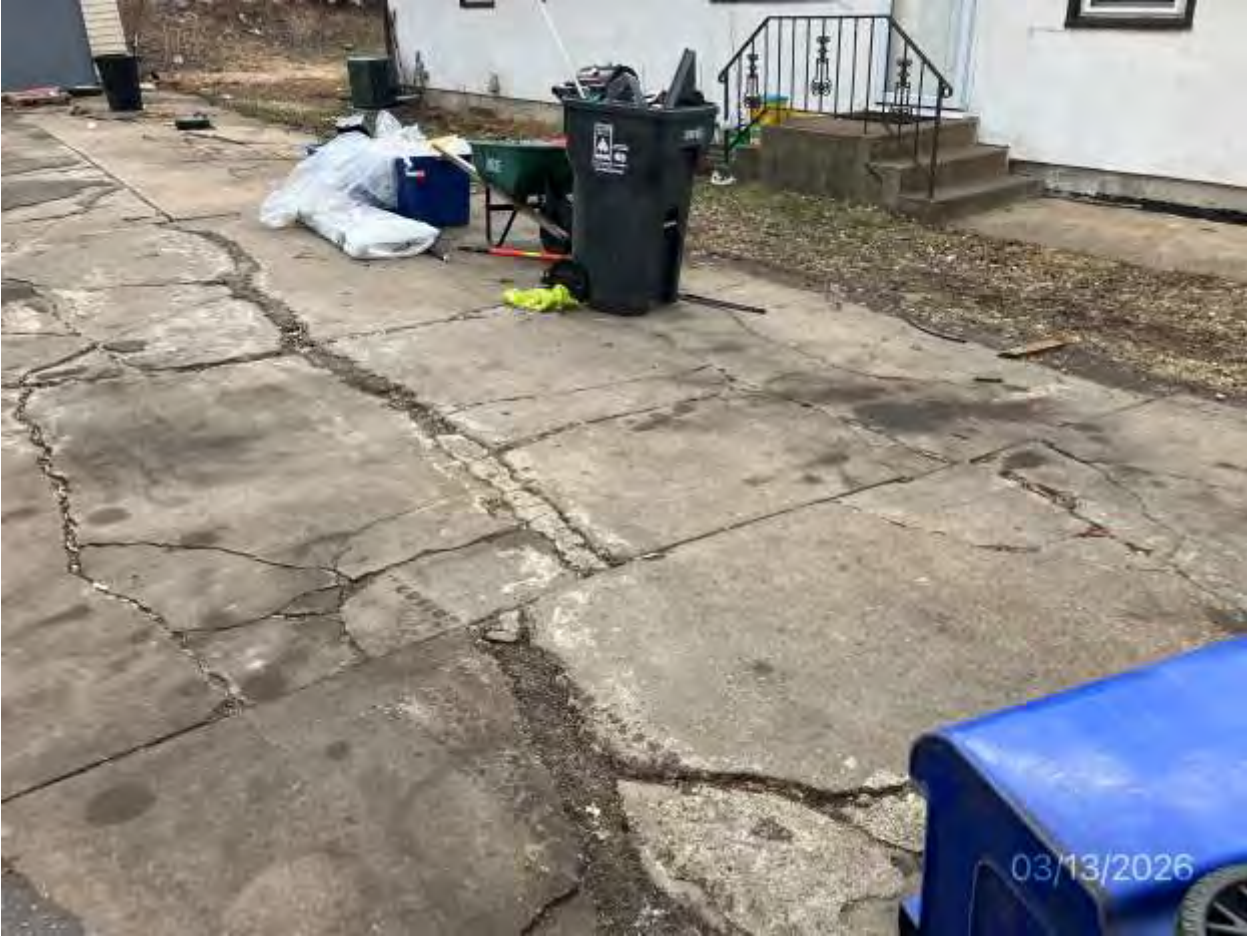
1164-1166 Cumberland St.Photos Before/After Clean Up 3-30-26
