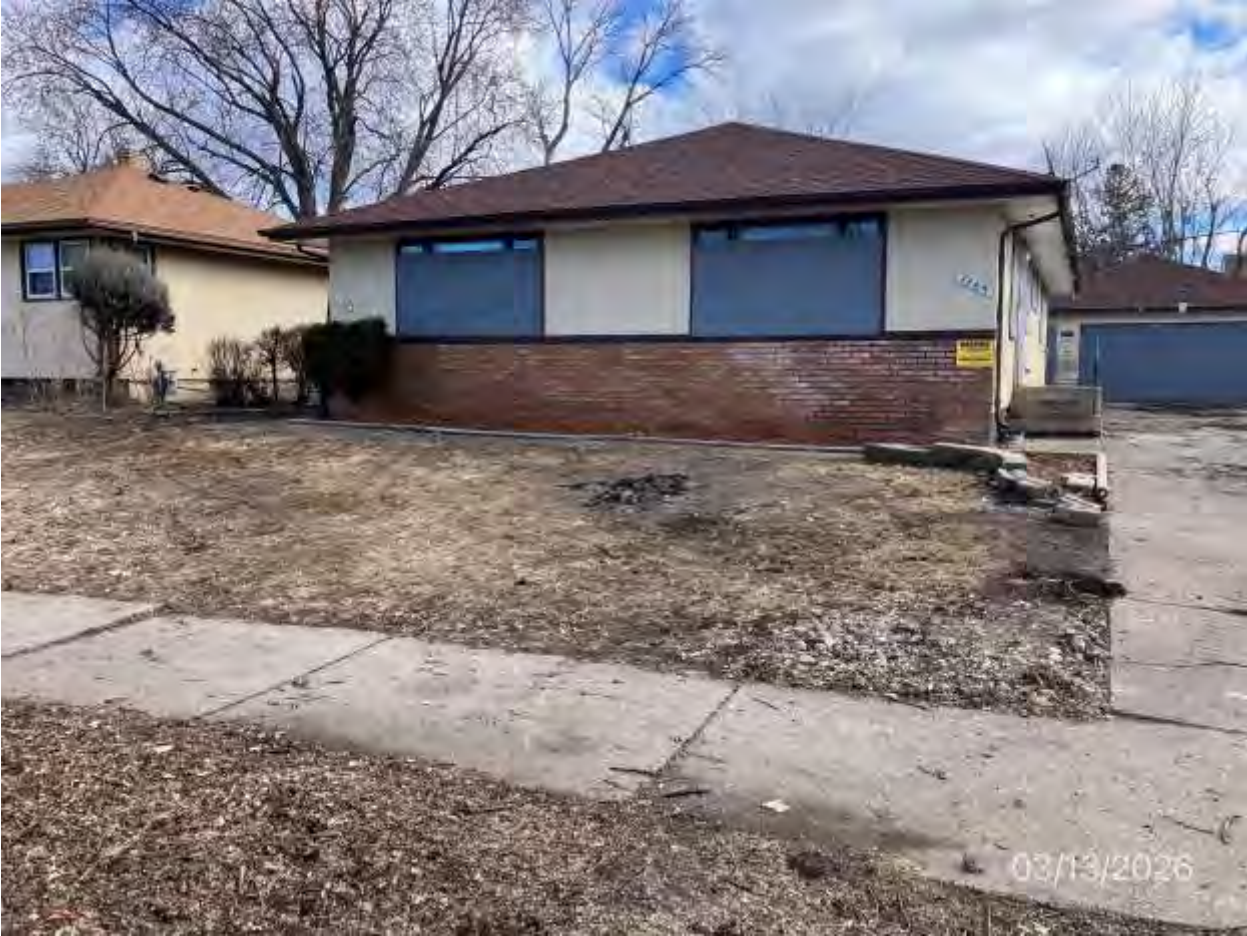
1164-1166 Cumberland St. Photos Before/After Clean Up 3-30-26
