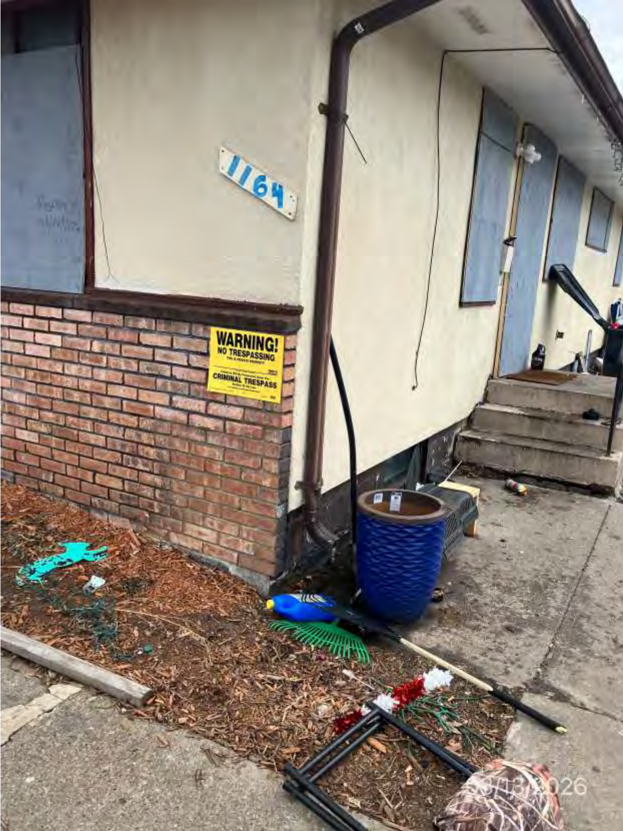
1164-1166 Cumberland St. Photos Before/After Clean Up 3-30-26
