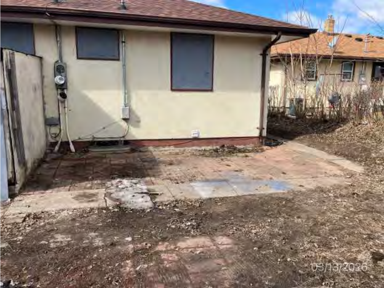
1164-1166 Cumberland St. Photos Before/After Clean Up 3-30-26
