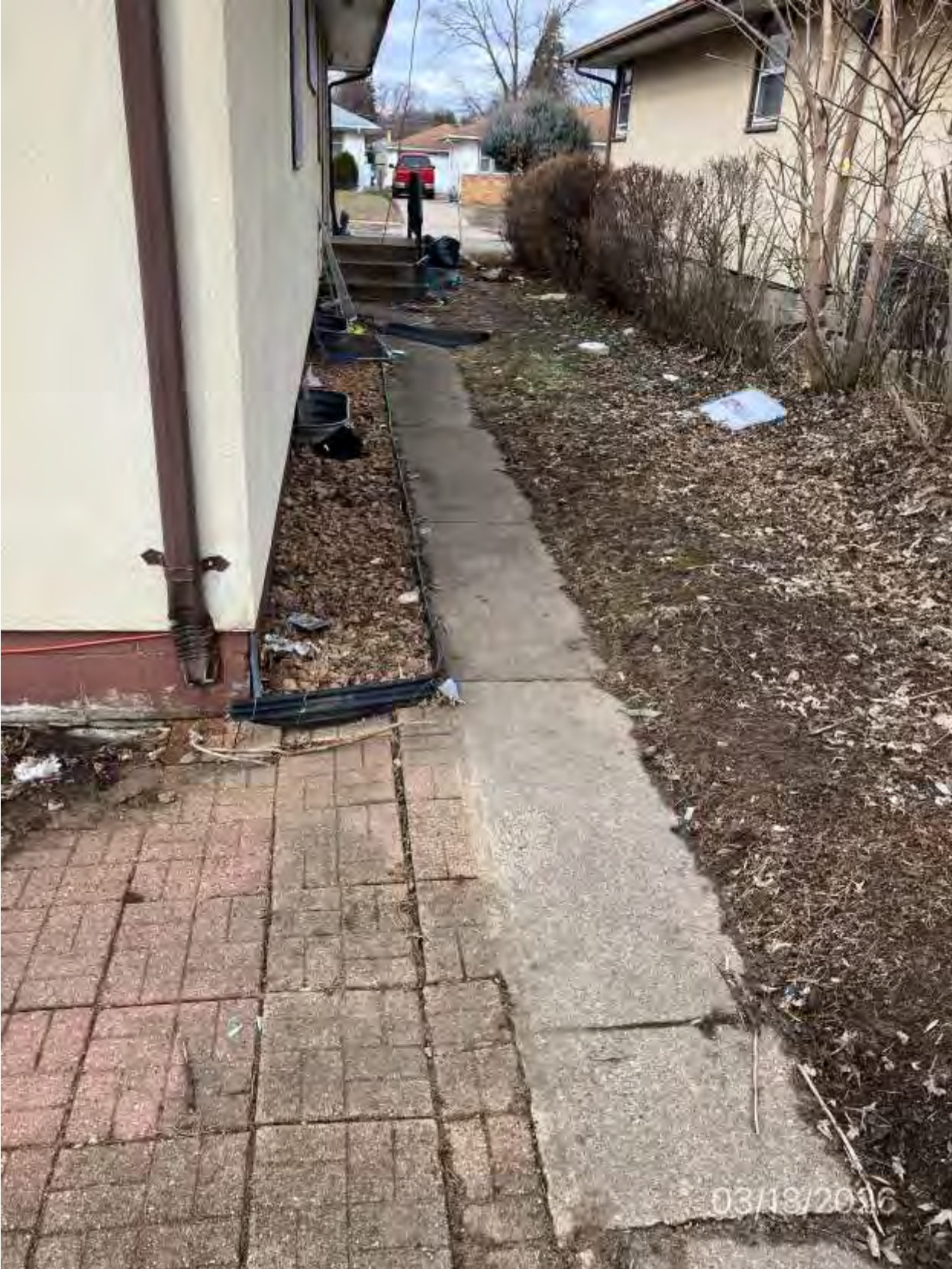
1164-1166 Cumberland St. Photos Before/After Clean Up 3-30-26
