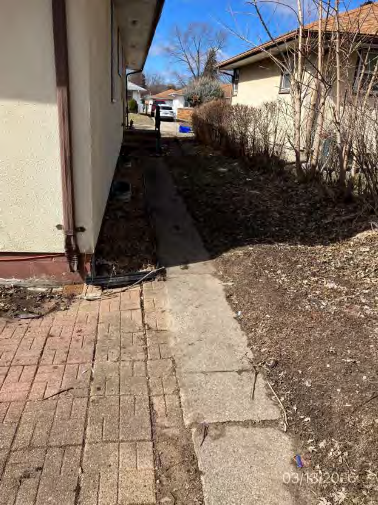
1164-1166 Cumberland St. Photos Before/After Clean Up 3-30-26
