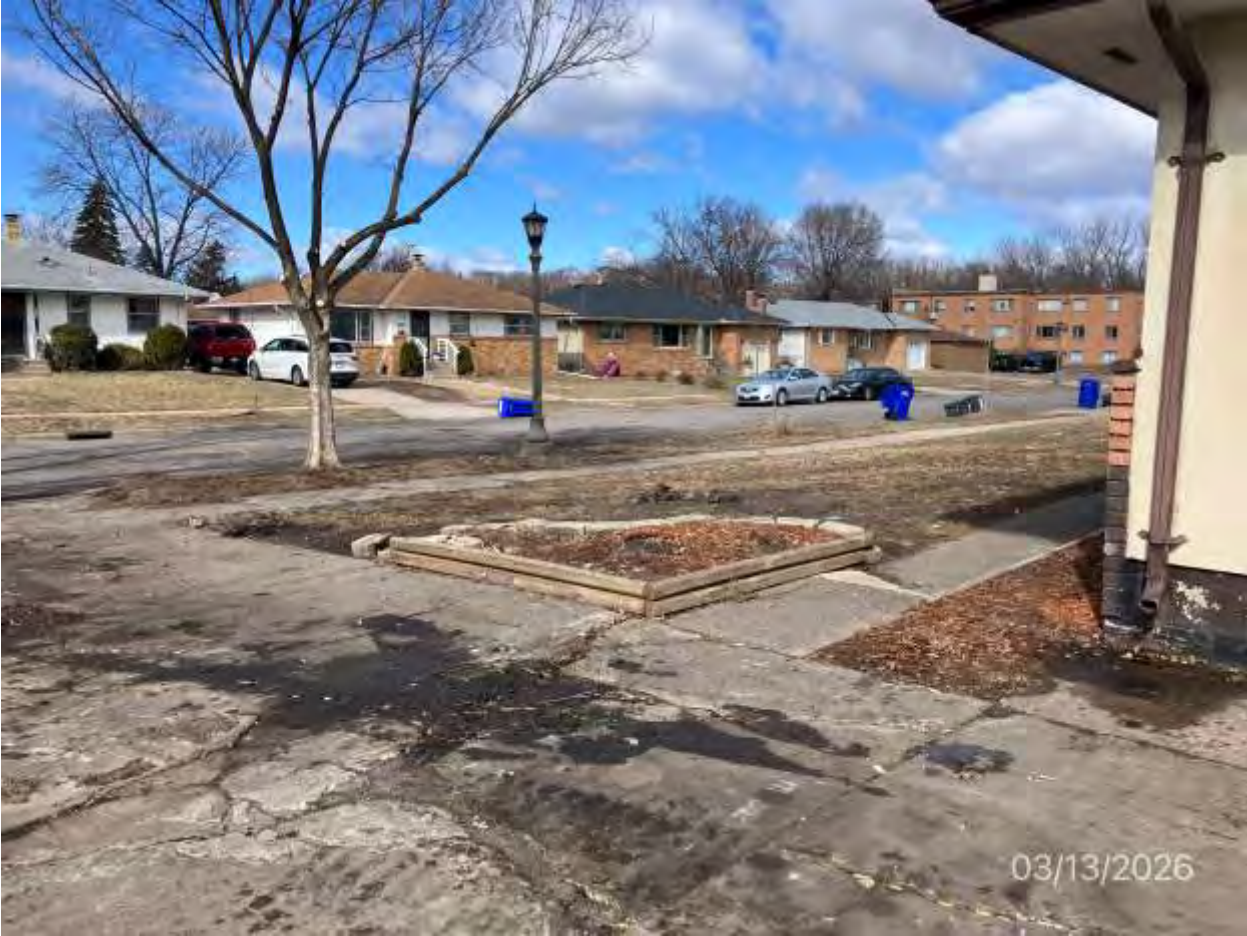
1164-1166 Cumberland St.Photos Before/After Clean Up 3-30-26
