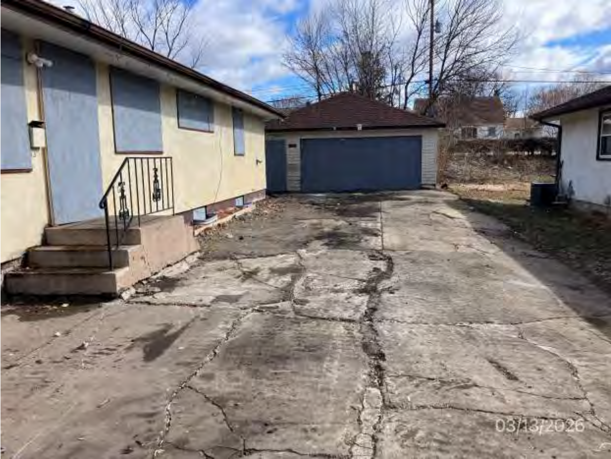
1164-1166 Cumberland St.Photos Before/After Clean Up 3-30-26
