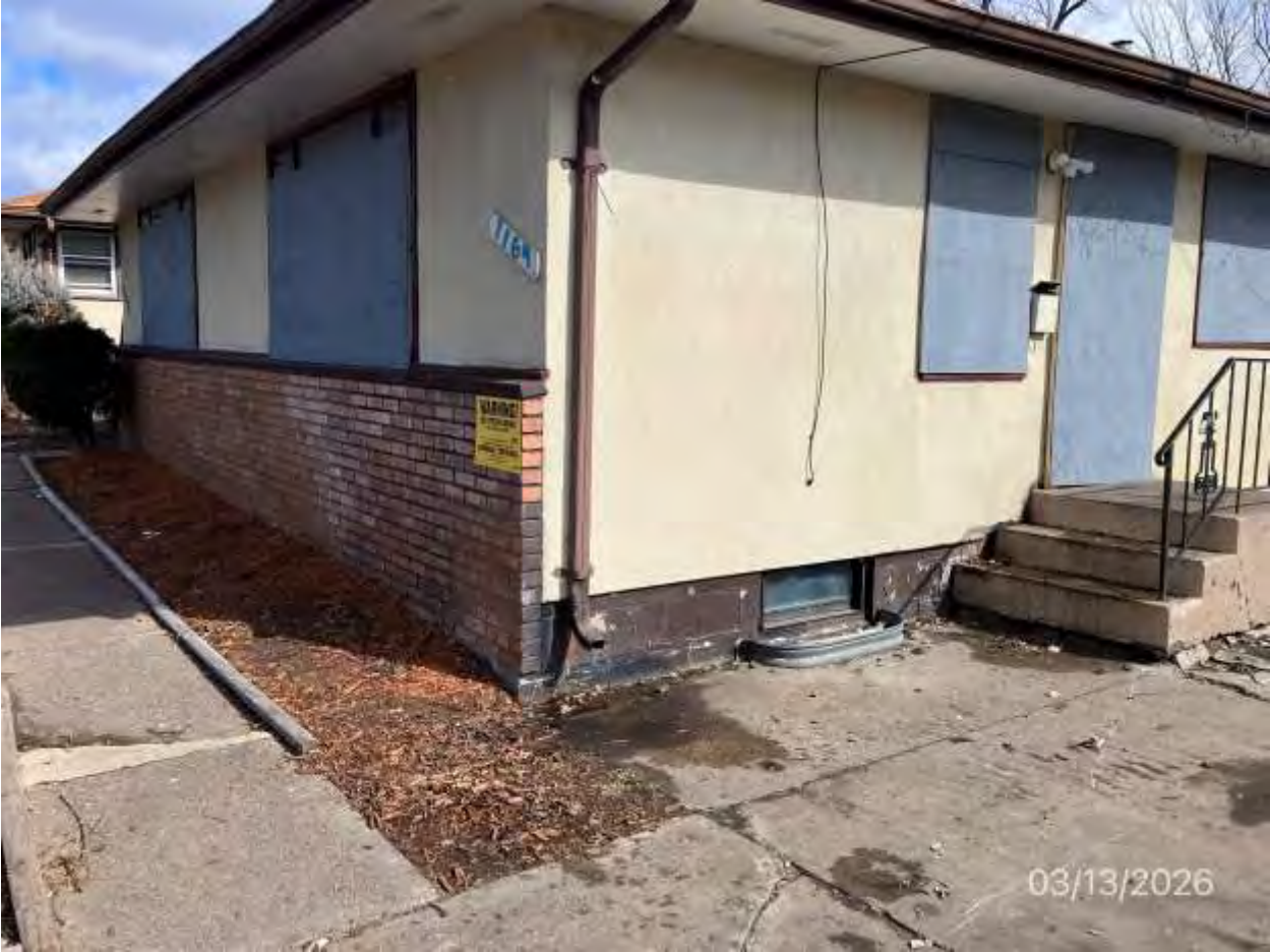
1164-1166 Cumberland St. Photos Before/After Clean Up 3-30-26
