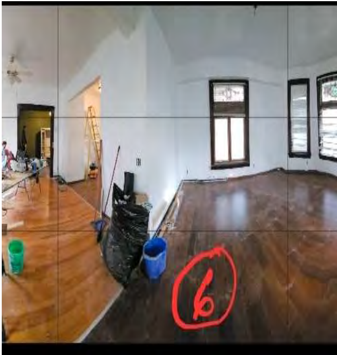
nrew floor in LR and stairs area & new paint
