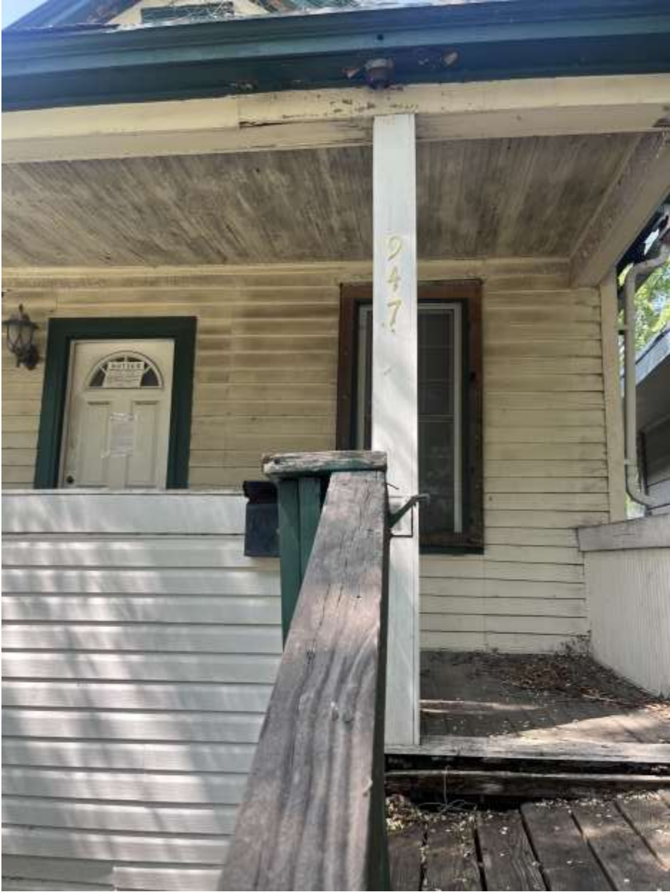
947 Fremont Ave.contractor photos 6-2-25
