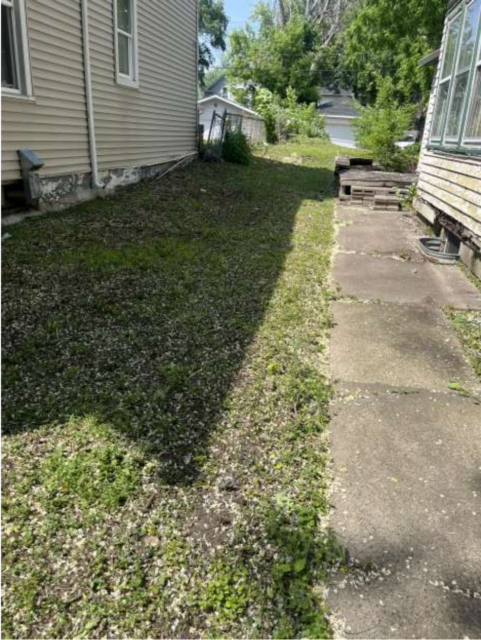
947 Fremont Ave.contractor photos 6-2-25
