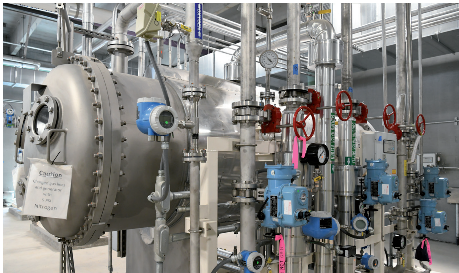
Ozonation equipment in the new water treatment plant on a tour May 9.
