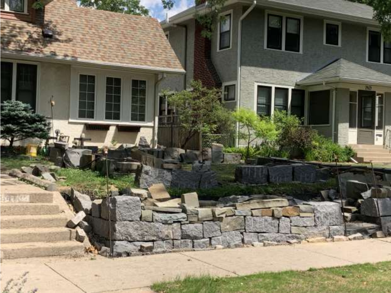
1473 Fairmount Ave. Retaining Wall 7-7-26
