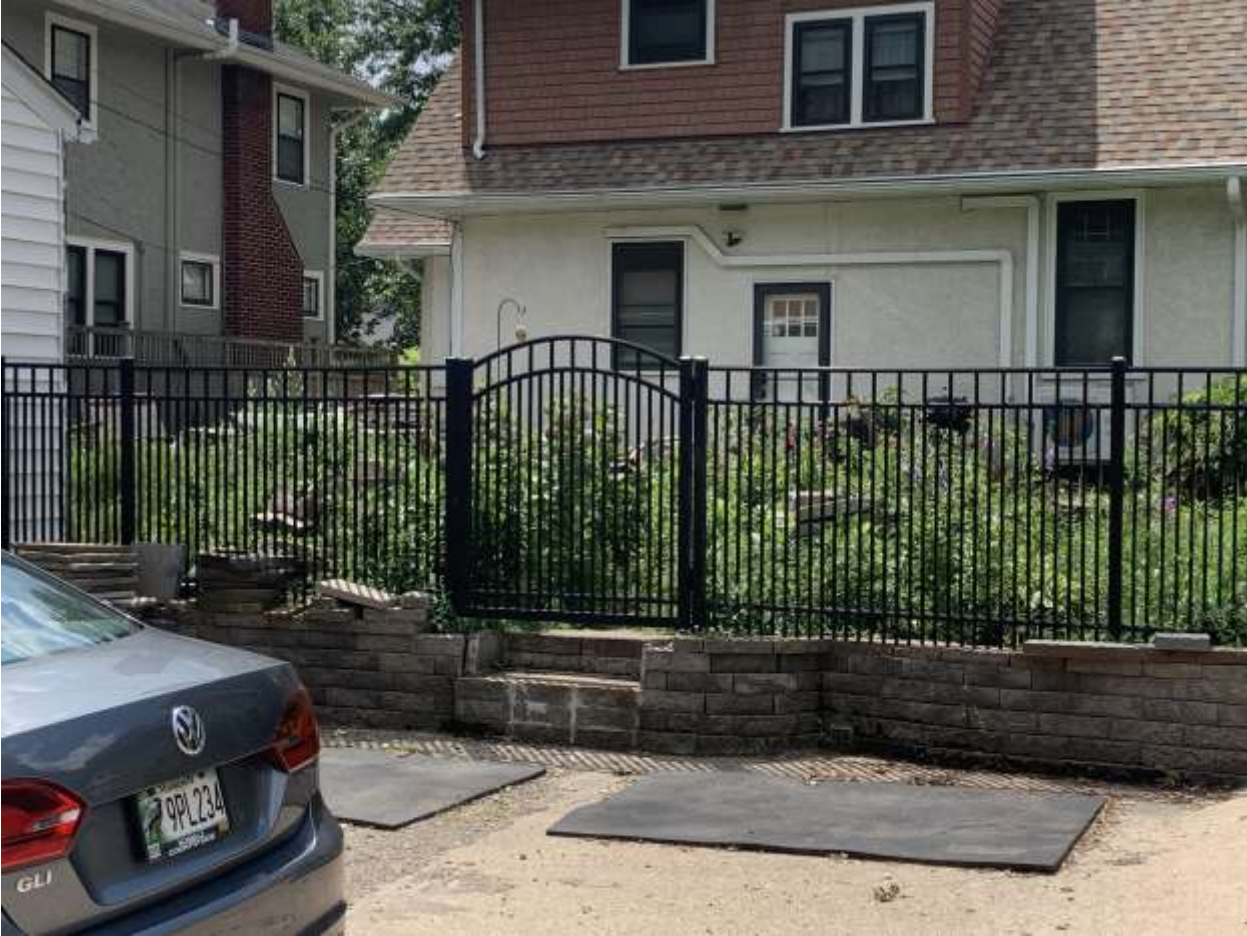
1473 Fairmount Ave.Retaining Wall 7-7-26
