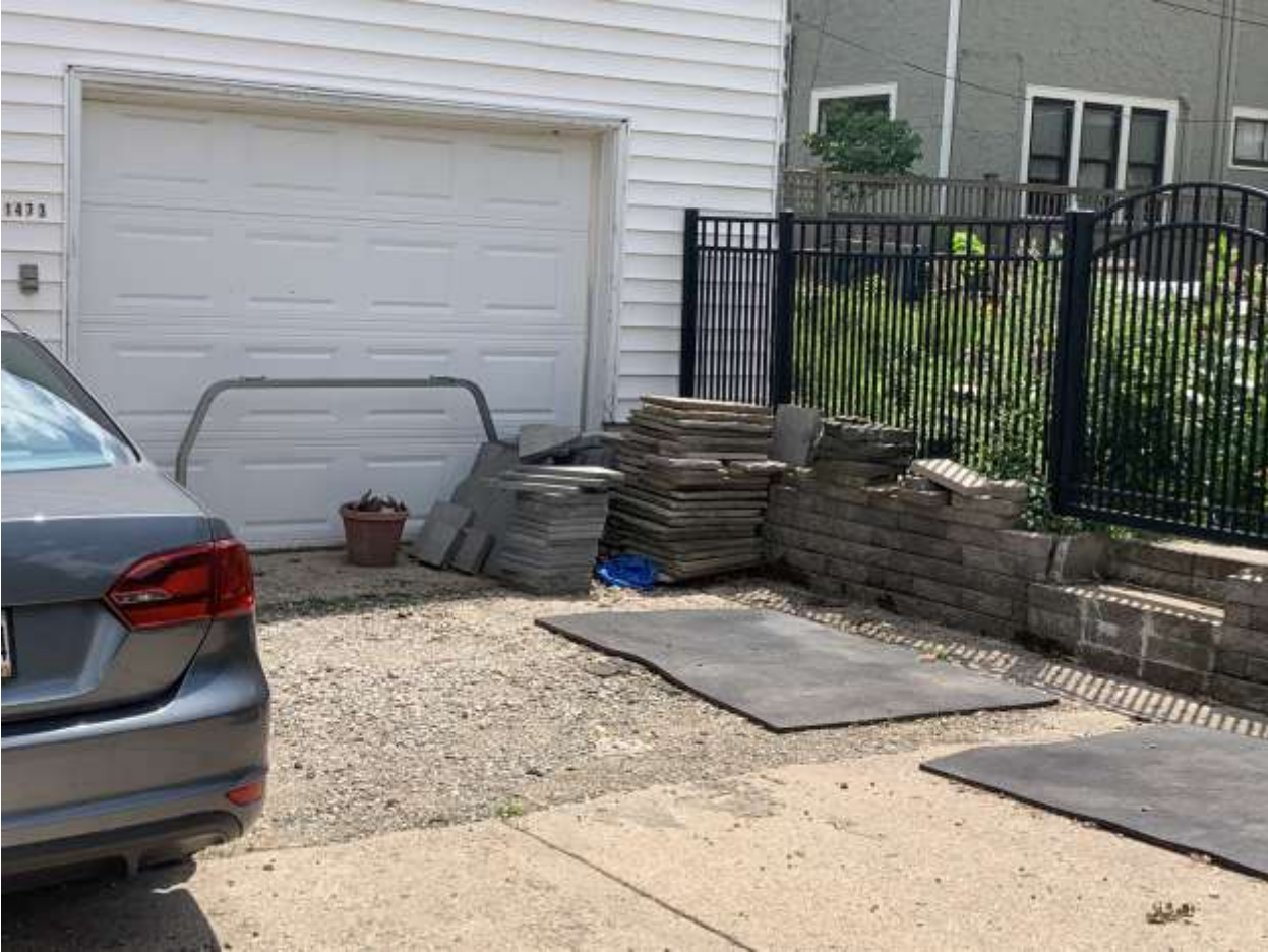
1473 Fairmount Ave. Retaining Wall 7-7-26
