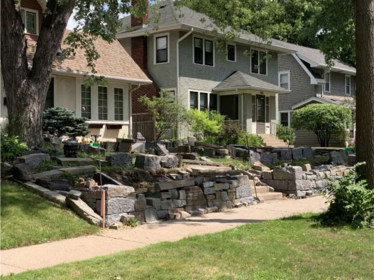
1473 Fairmount Ave.Retaining Wall 7-7-26
