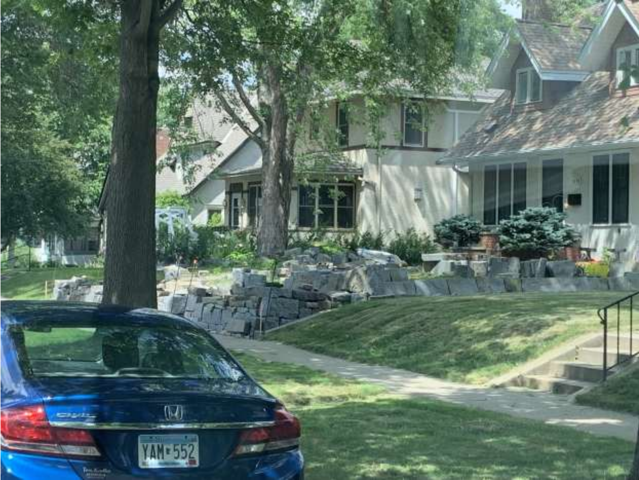
1473 Fairmount Ave. Retaining Wall 7-7-26
