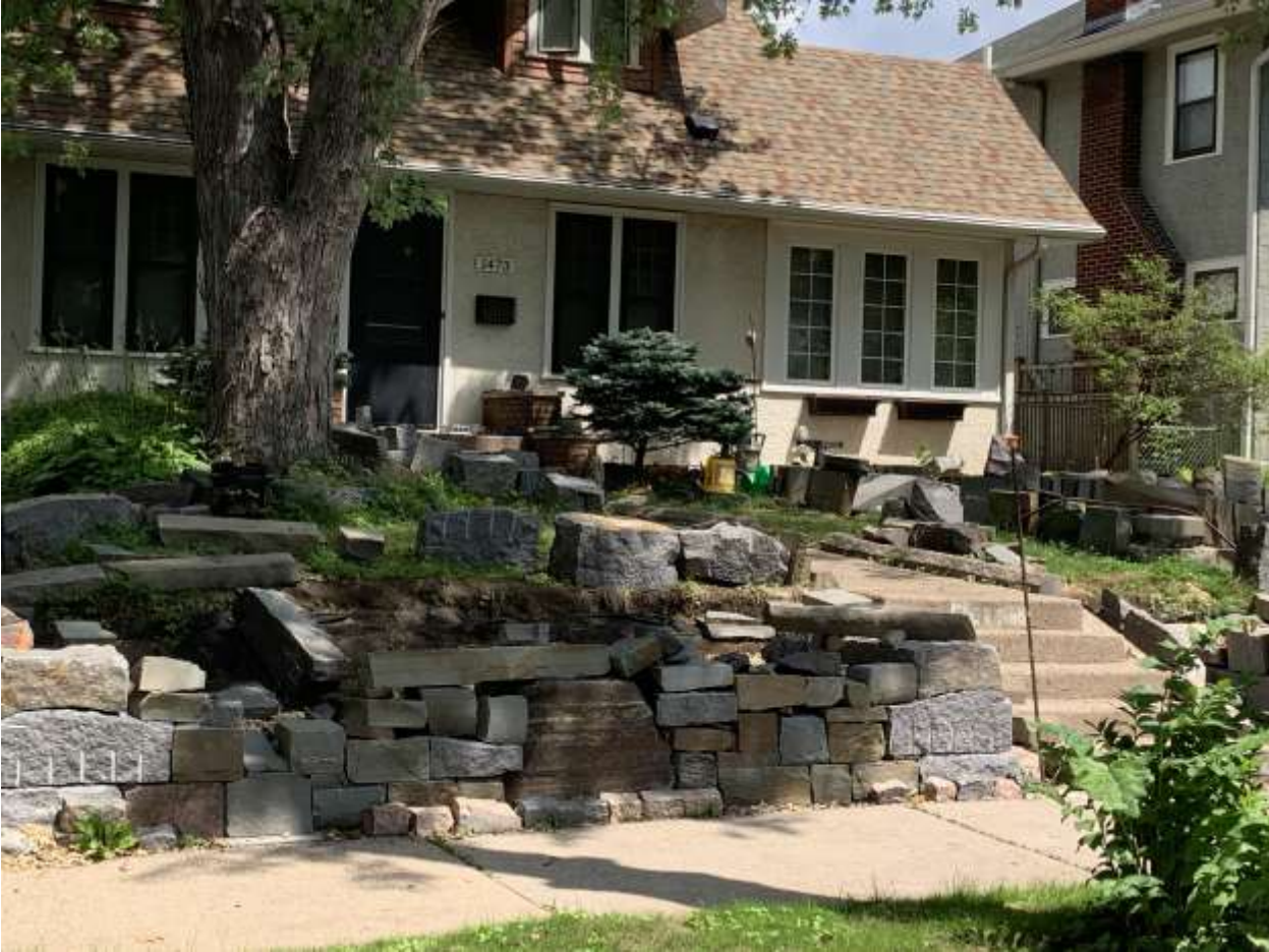
1473 Fairmount Ave.Retaining Wall 7-7-26
