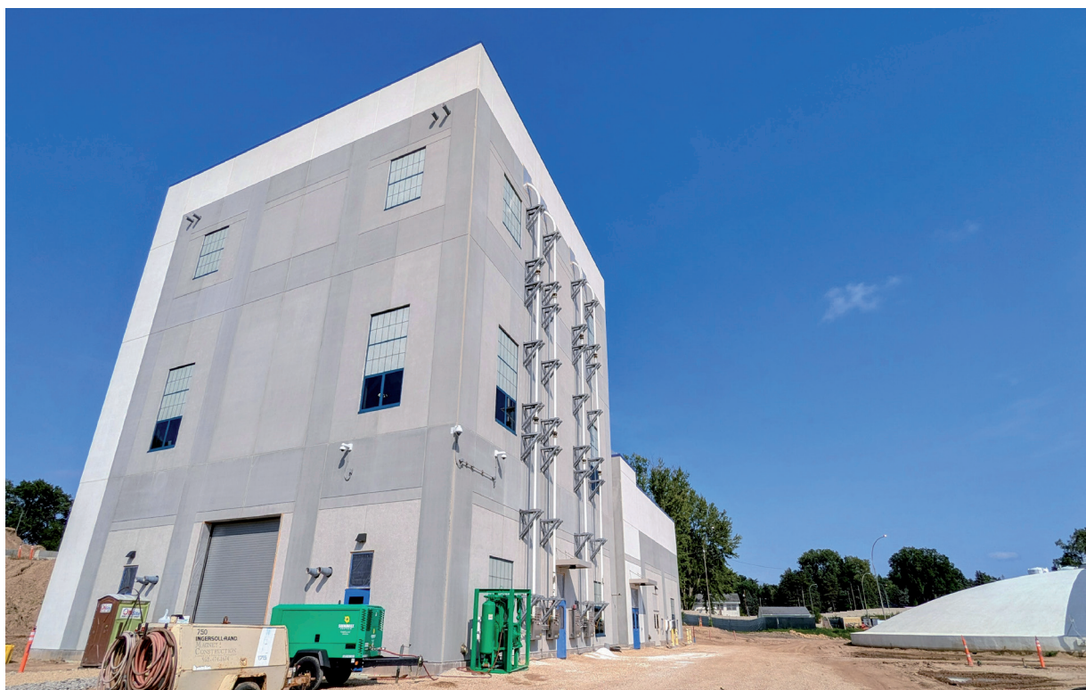
The new lime building towers over the tops of the clarifier domes to the right at the new treatment plant.
