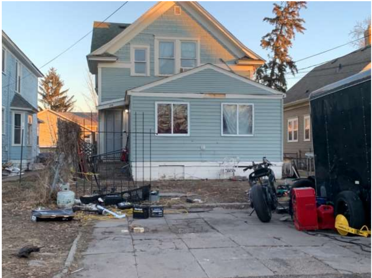
650 Lafond Ave. photo from SAO 1-6-25
