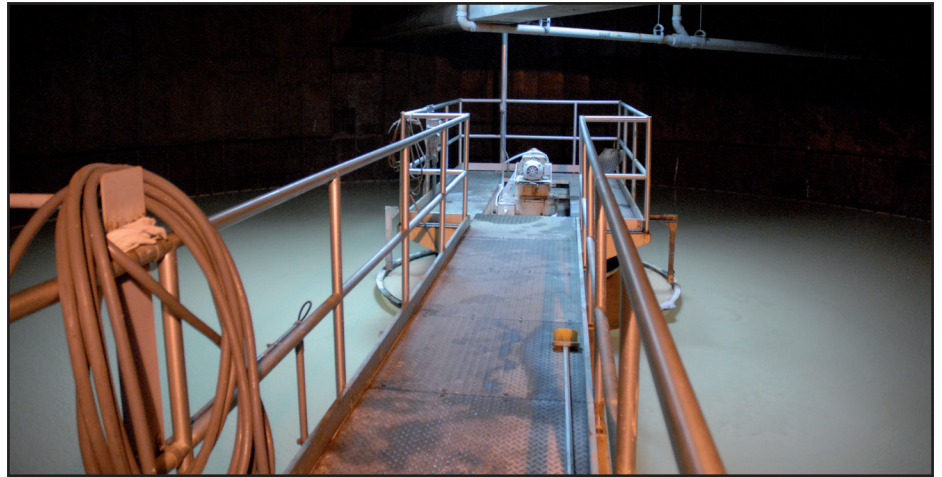
Sludge goes to the thickener to reduce the amount of liquid in the sludge.
