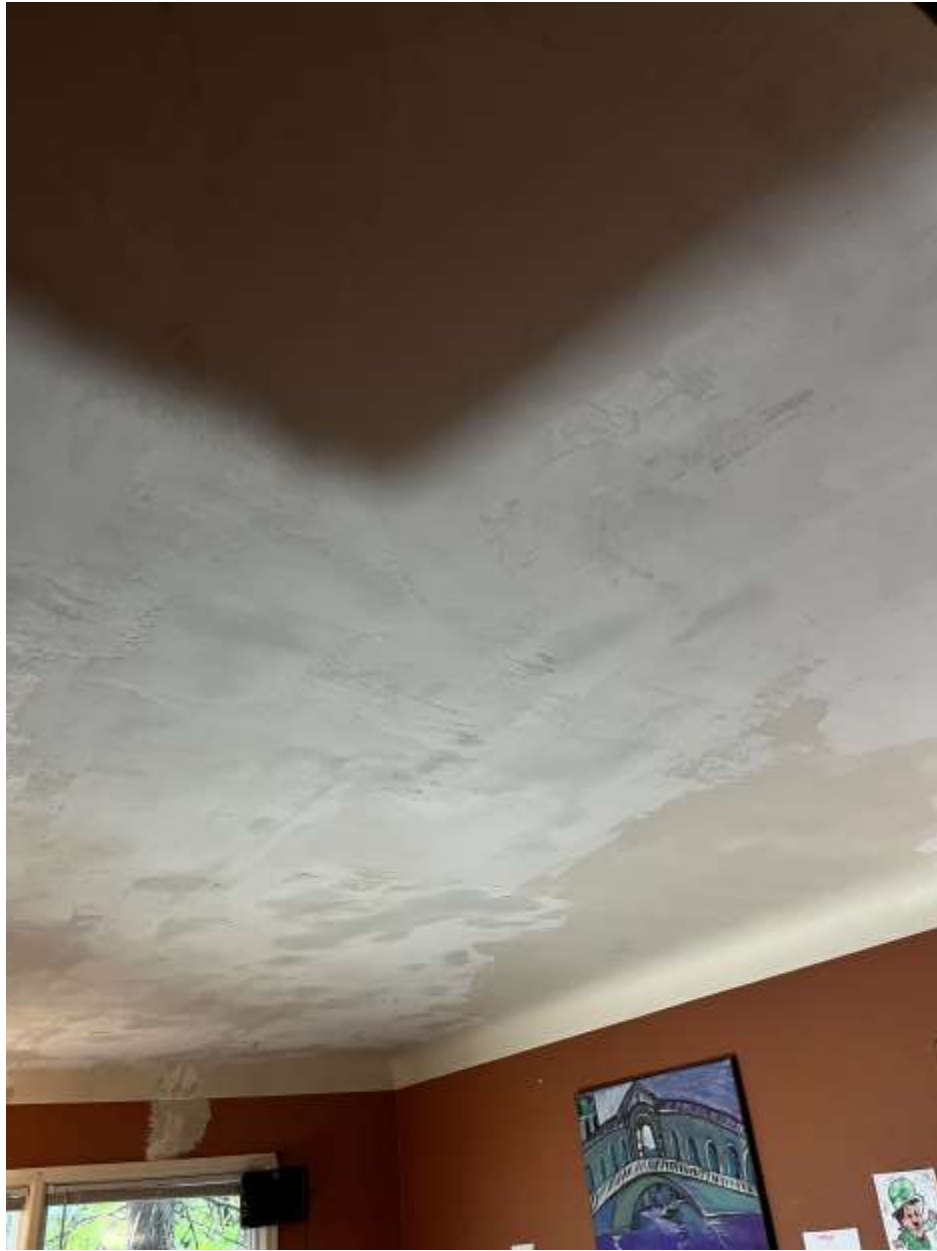
1220 Sherburne Ave. repair photos by Valmyr 5-20-25
