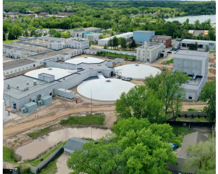
The new clarifiers at the new treatment plant.
