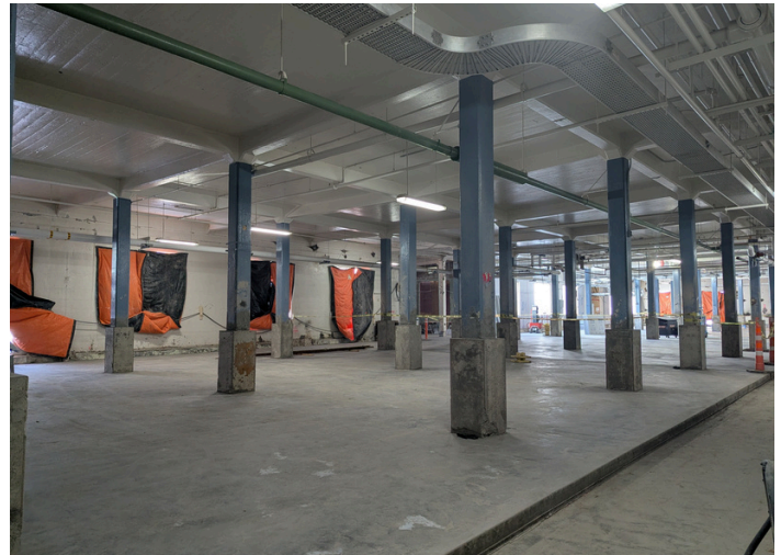
Floc 2 after the floor was created using concrete.
