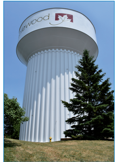
Cope Avenue tank in Maplewood.
