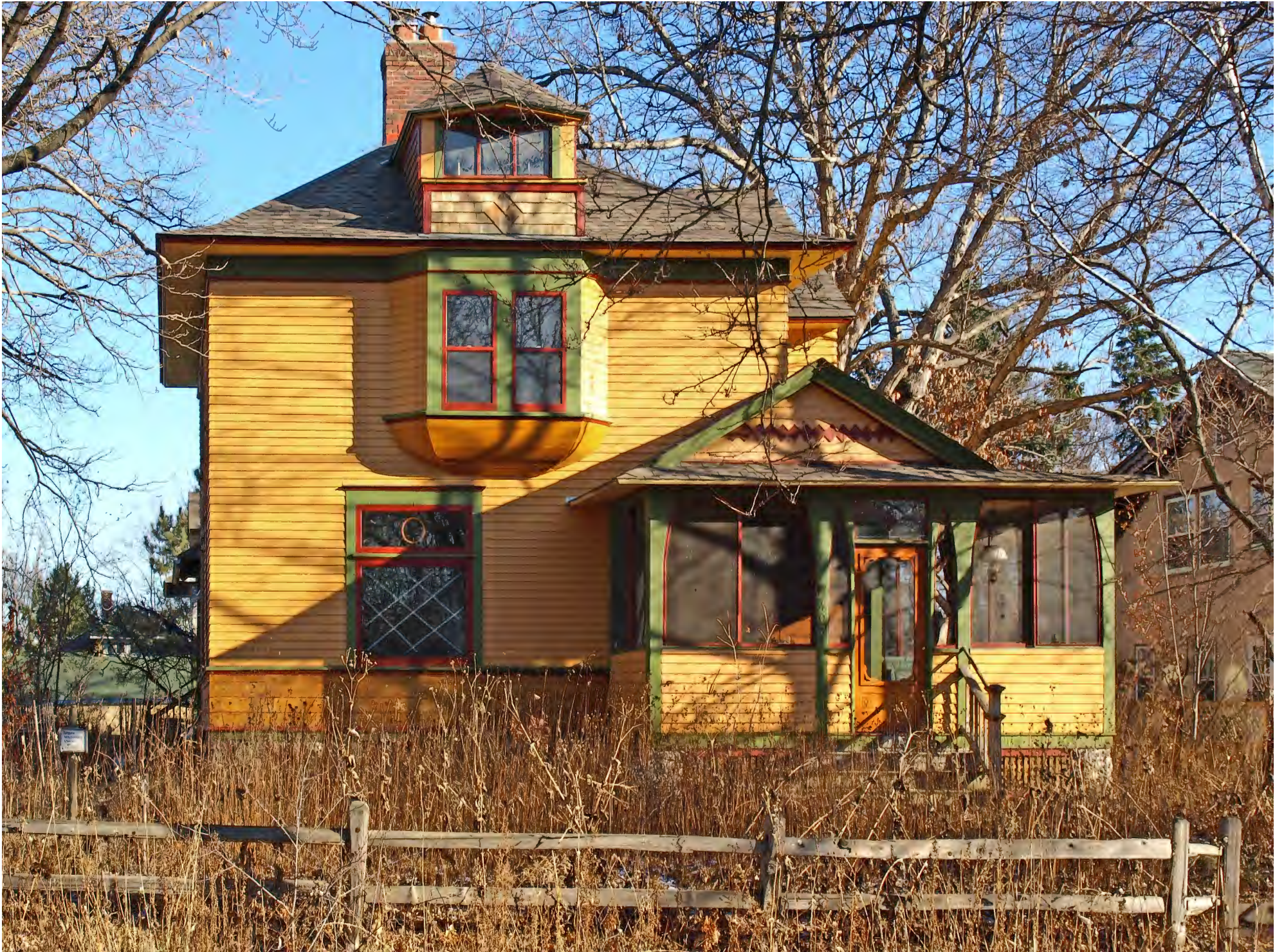
Dwight and Clara Watson House_0001 house viewed from west, west elevation, camera facing east
