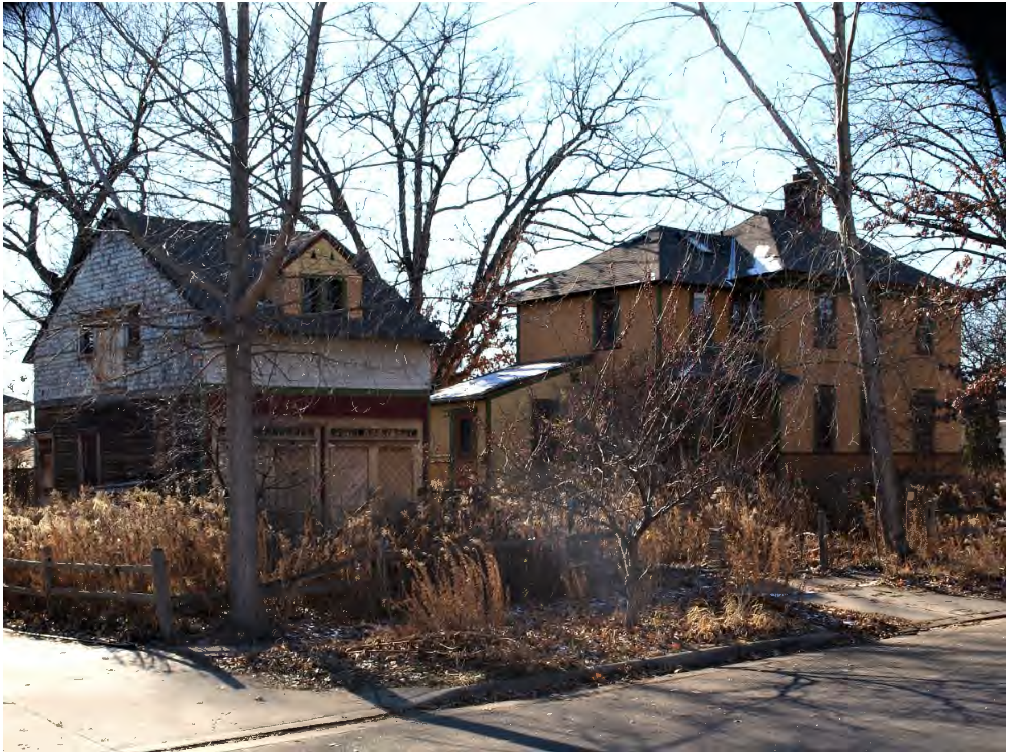
Dwight and Clara Watson House_000 barn and house on Delos tree viewed from northeast, east and north elevations, camera facing southwest
