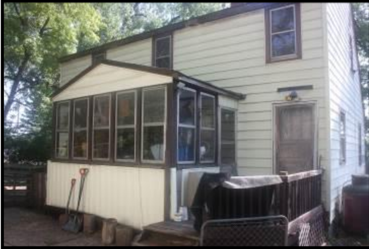
Rear view-west elevation
