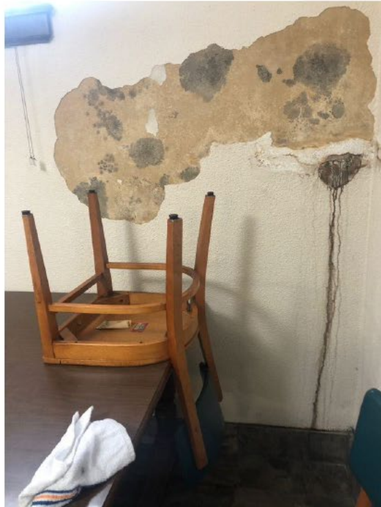
Water damage in community room
