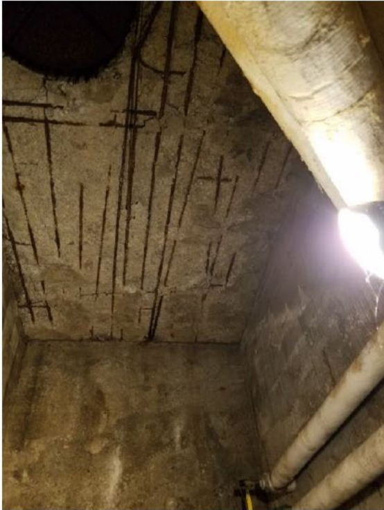
Exposed rebar and spalling concrete
