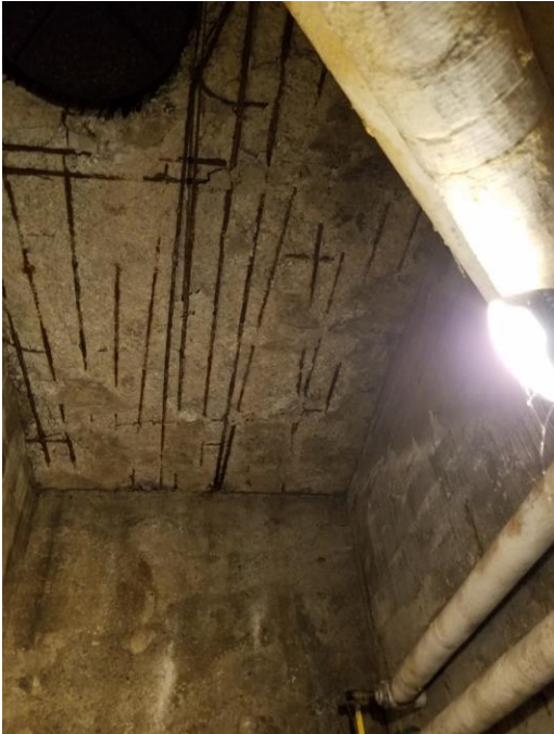
Exposed rebar and spalling concrete
