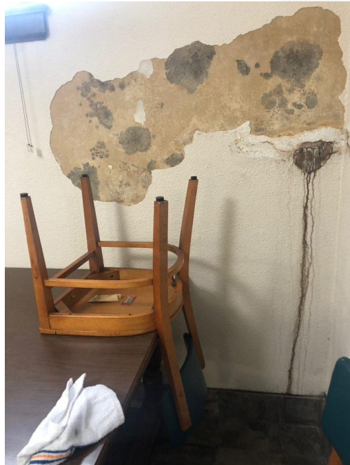
Water damage in community room
