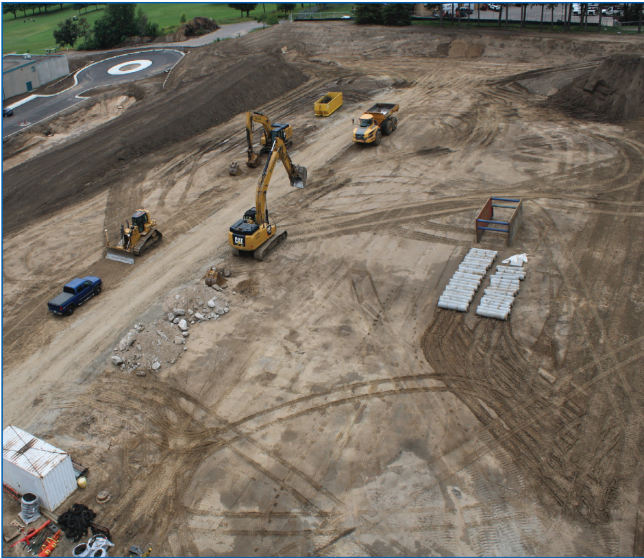
The Highland reservoir, located south of the water tower on Snelling Ave. is being demoed. The structure has been completely knocked down with the site being leveled. Note the new parking lot and cul de sac completed in front of the ice arena in upper left corner of the photo. Work continues on the reservoir as of August 27.
