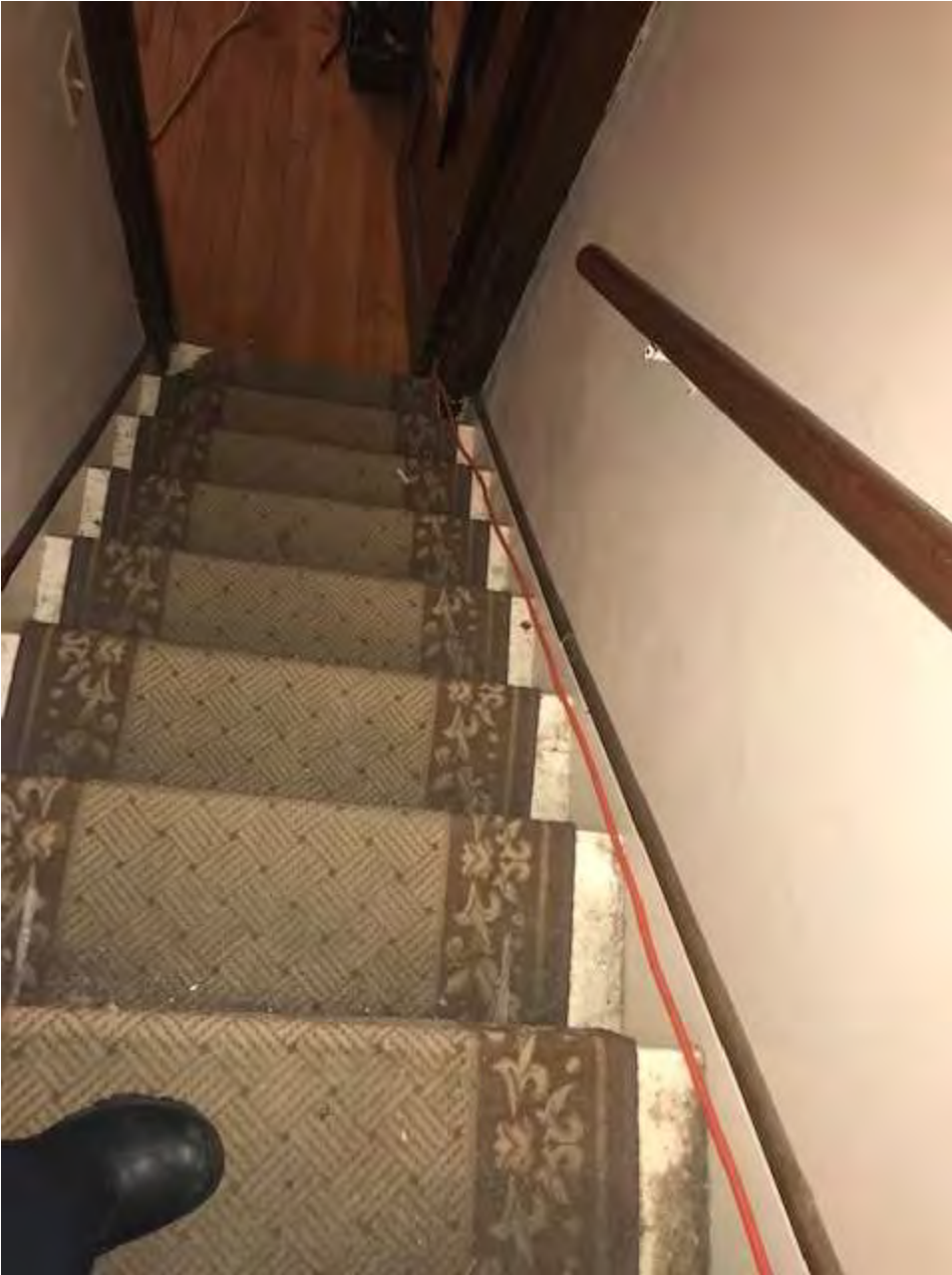
Stairway to top floor
