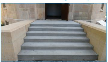
Renovation work to the Highland Park water tower was largely completed over the summer. Here the Kasota/Minnesota stone used for the entryway stairs on the north side is shown completely replaced. The stone on the west side of the tower was completely replaced as well, as were the doors at both entrances. More photos page 2.
