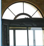
The arched window above the stairwell was set to be replaced along with the wooden framework, which had rotted out over time.
