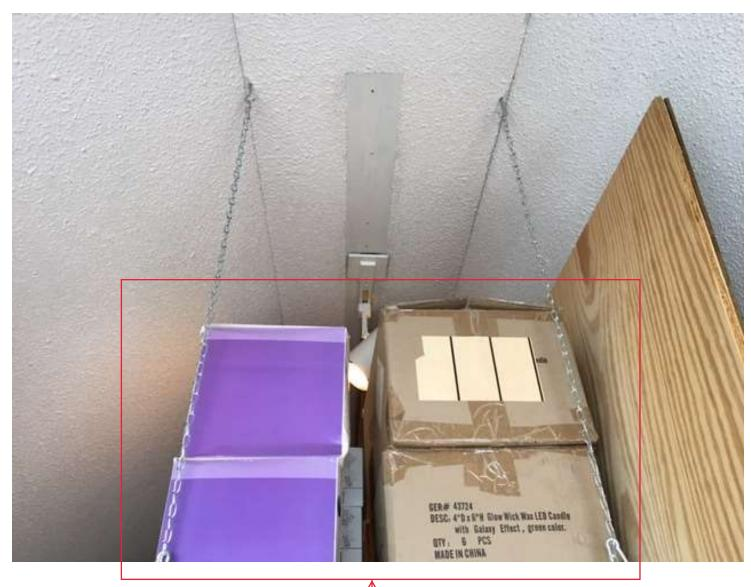
Storage is within 2 feet of the ceiling and must be removed.
