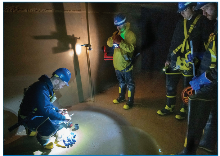
Andrew Magdziarz, maintenance worker, cleans out a check valve for the post finished water reservoir sample line deep within the south finished water reservoir on March 23. Tommy Hehn, water utility worker, shines a light on the work, with some assistance from Rich Hibbard, civil engineer. Rich and Tom Jauquet, civil engineer, were in the reservoir to take internal measurements since the reservoir was open for maintenance and repairs.
