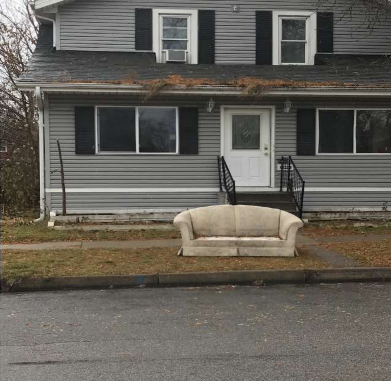
1048 Central Ave W Photos.11-22-19
