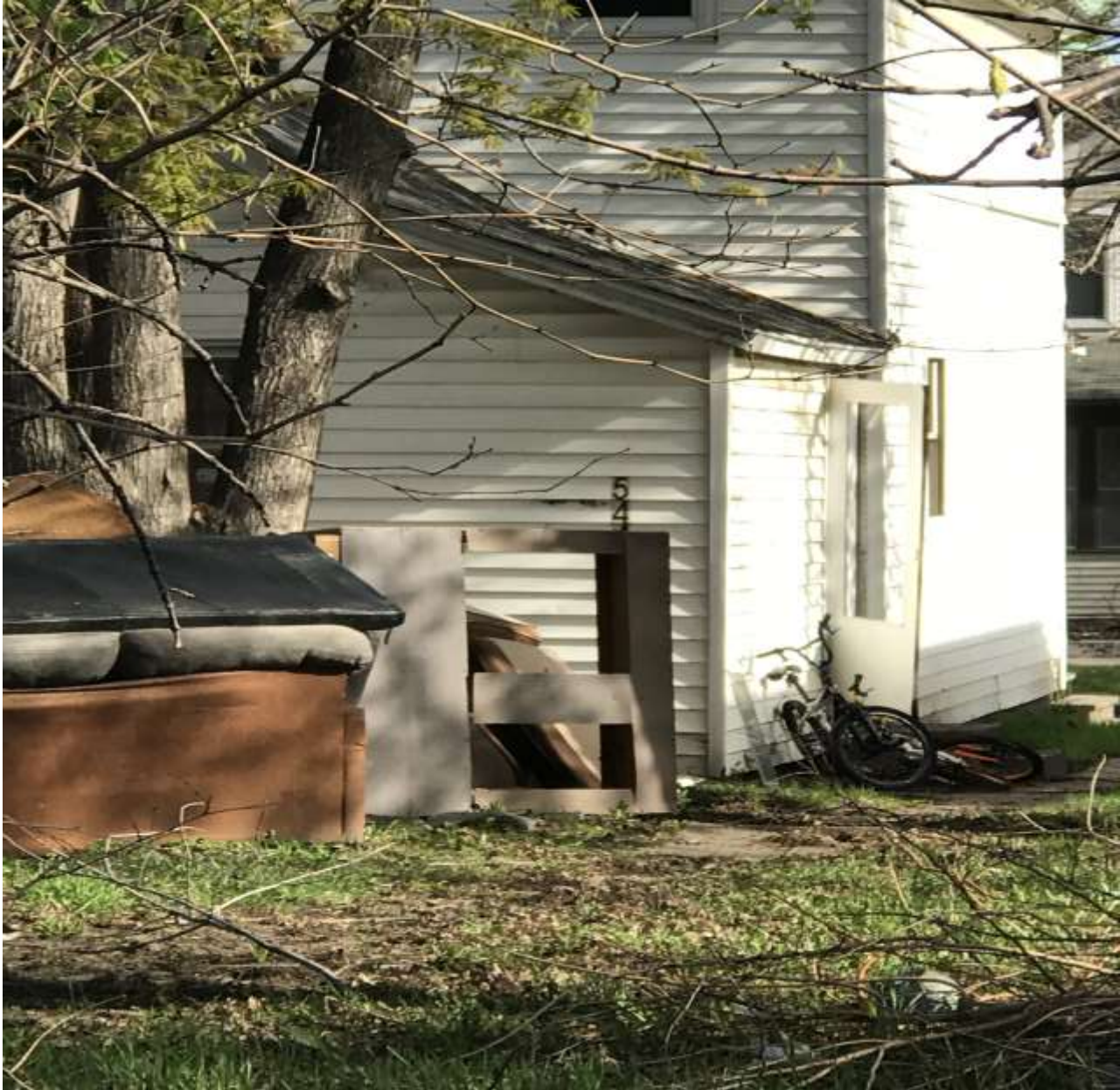
544 Sherburne Ave Photos taken 5/7/19
