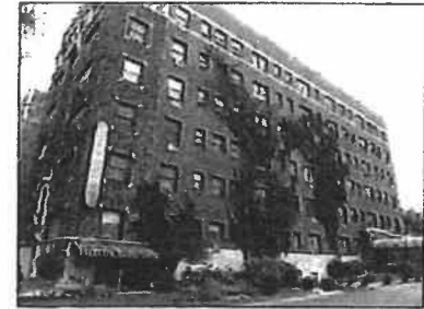
NORTHEASTERLY CORNER OF COMMODORE APARTMENT BUILDING
