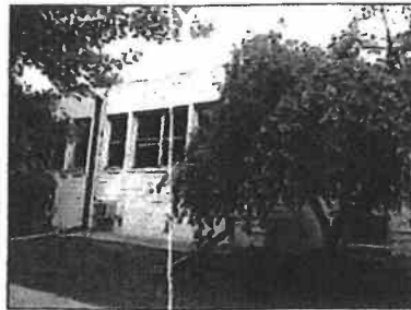
SOUTHERLY OUTSIDE BUILDING WALL OF PROPOSED BANQUET ROOM PARCEL
