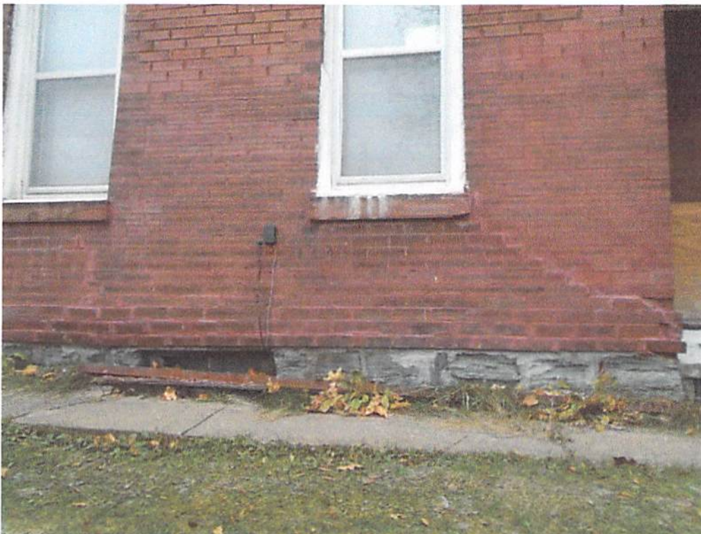
Photo 2: Another photo of the north wall in question, with stair step cracking starting at the sill of from the westernmost window.
