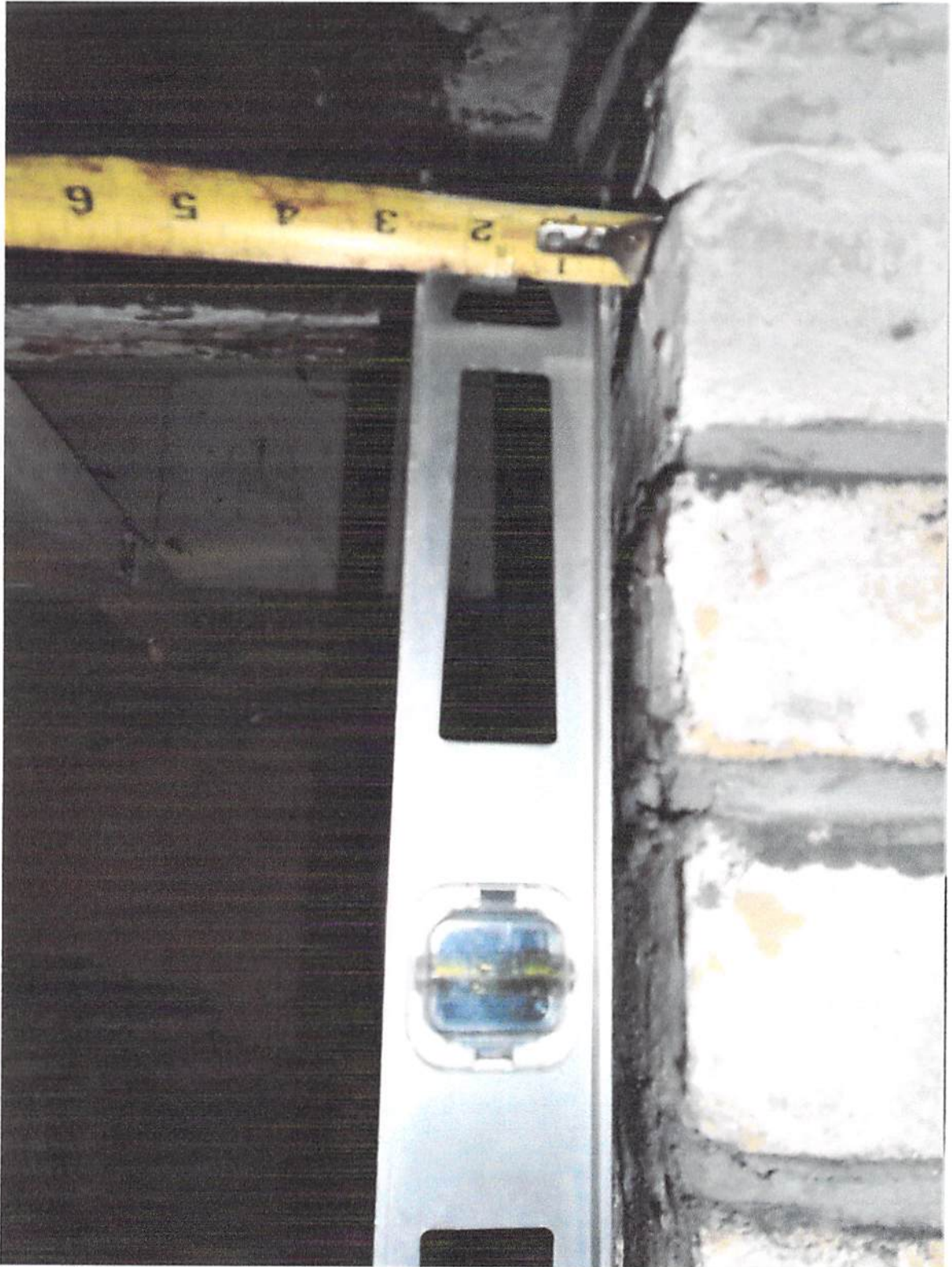
Photo 10: Measurement of the plumbness of the foundation wall west of the basement window on the north side of the residence.
