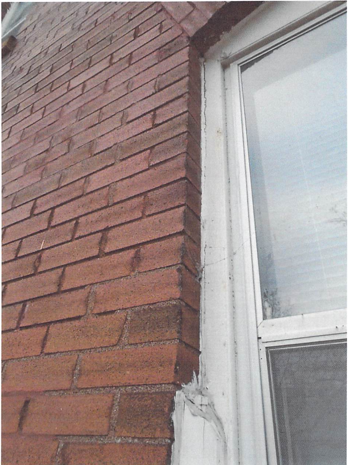
Photo 3: Deteriorated sealant on wood molding around perimeter of window stops show of window head.
