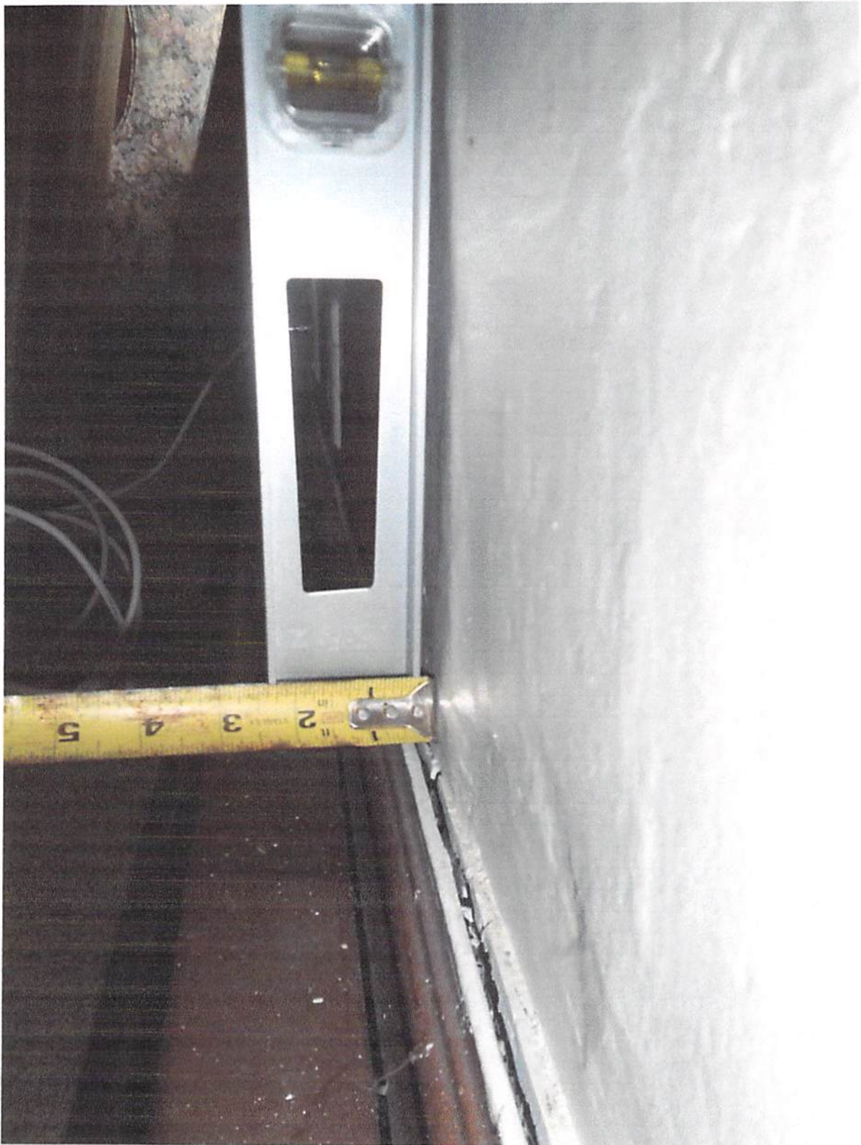
Photo 11: Inside face of interior wall behind the brick façade along the north wall was out of plumb a little less than \frac{1}{4} " in 4ft.
