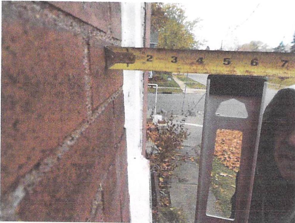
Photo 7: The north wall east of the window opening was approximately 4\frac{3}{16} " out of plumb in 4ft.
