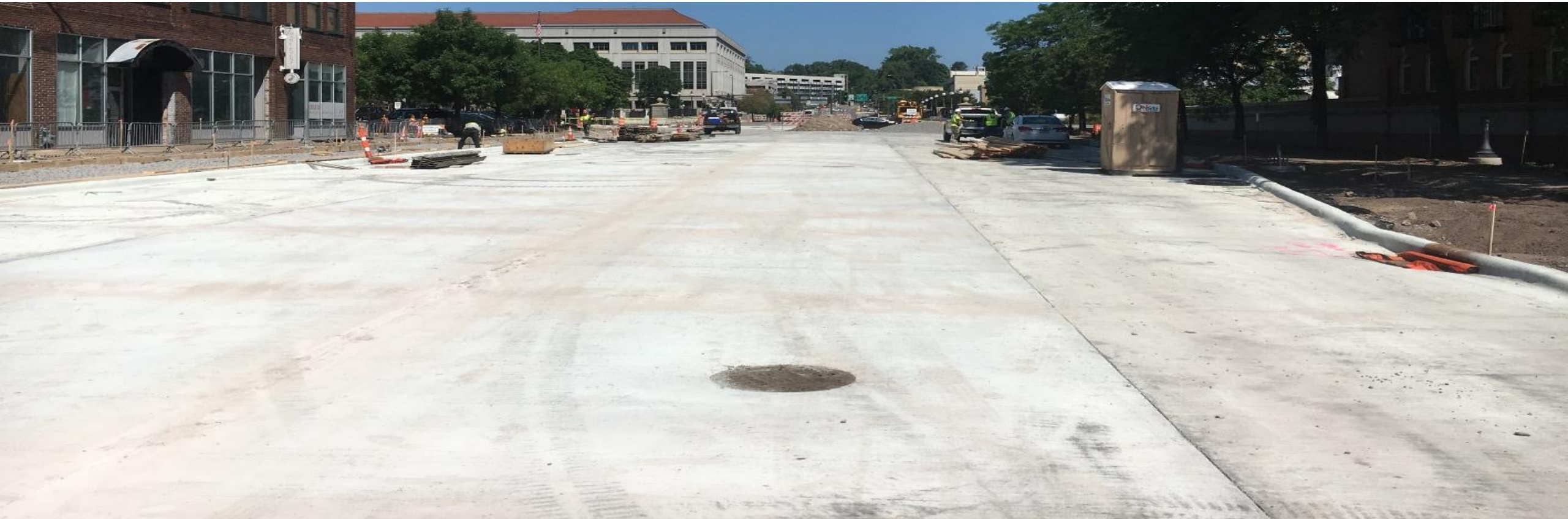
The Jackson Street Reconstruction Project
