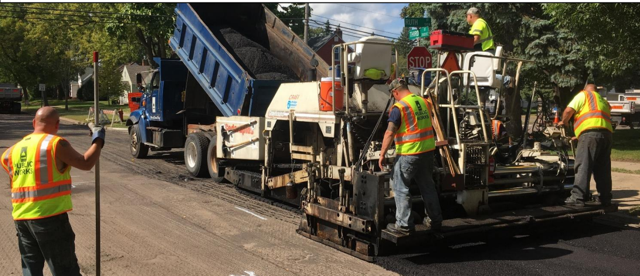
Mill and Overlay
