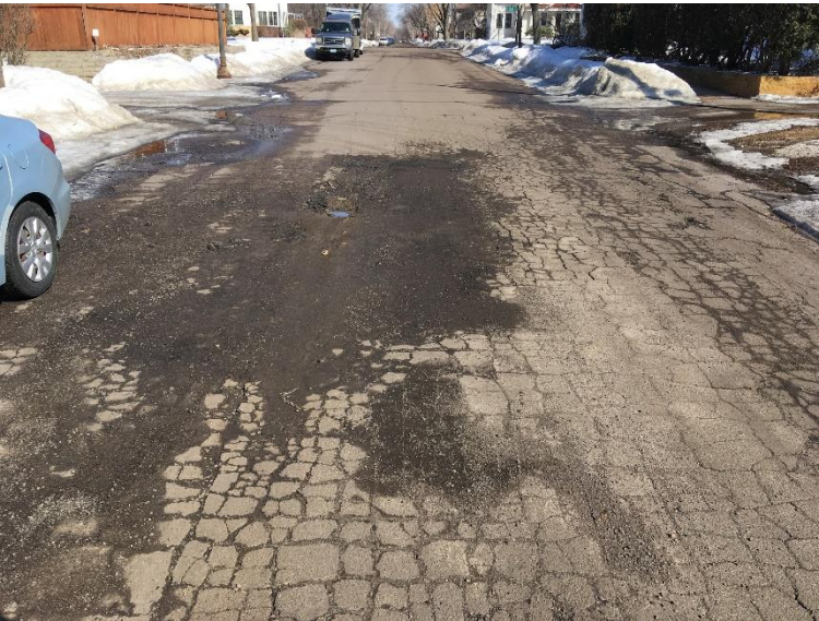
PCI = 40 (Poor)
