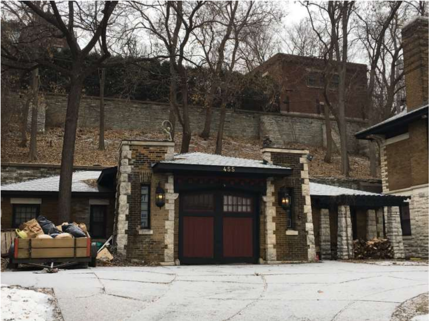
Front of the carriage house
