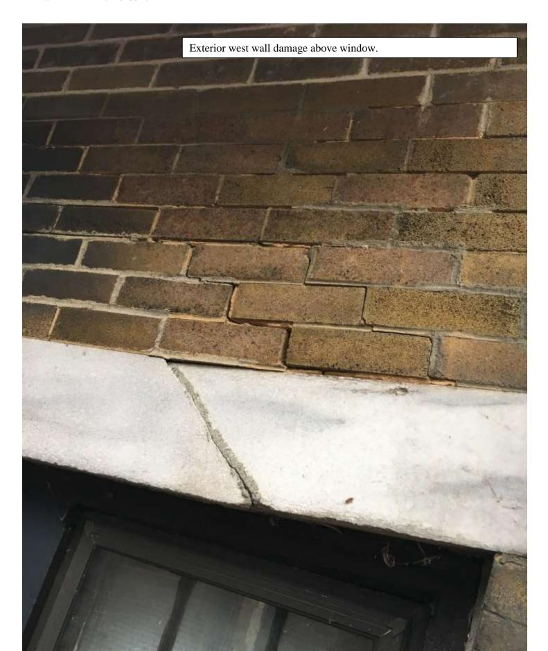
More damage exterior west wall. Window pulling away from the brick
