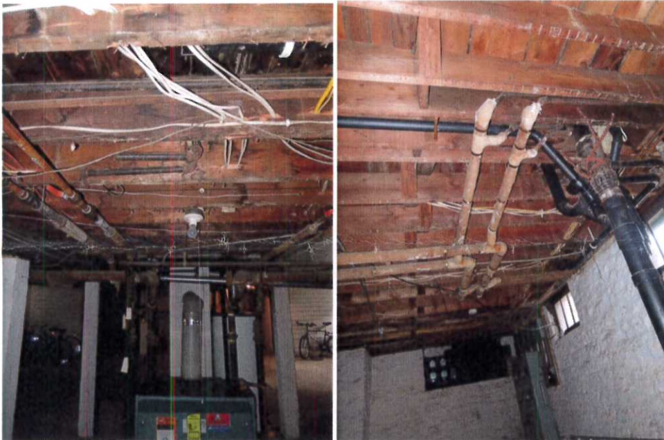
Pictures of basement ceiling at 1725 Hague Ave., Saint Paul
