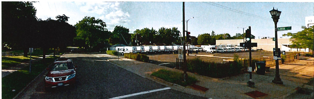
Albion Street with Post Office to the east of the project site
