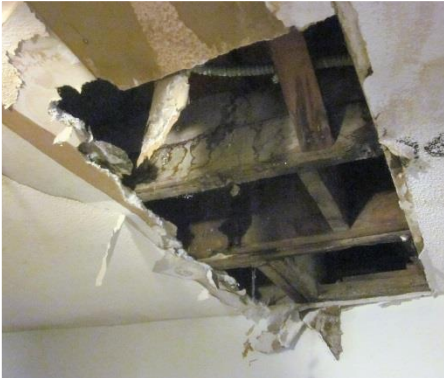
Leaking Ceiling
