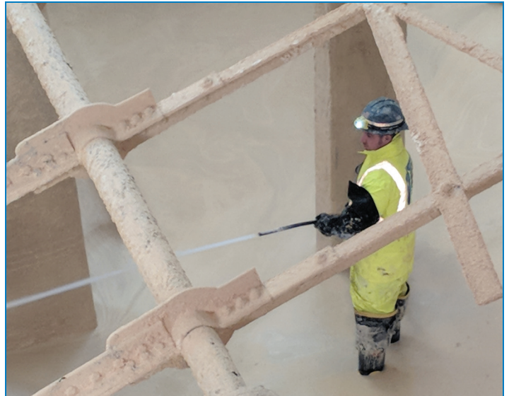
Herman Audett, water utility worker, begins clean out of flocc 3, which also needed repairs, during its annual maintenance Jan. 5.
