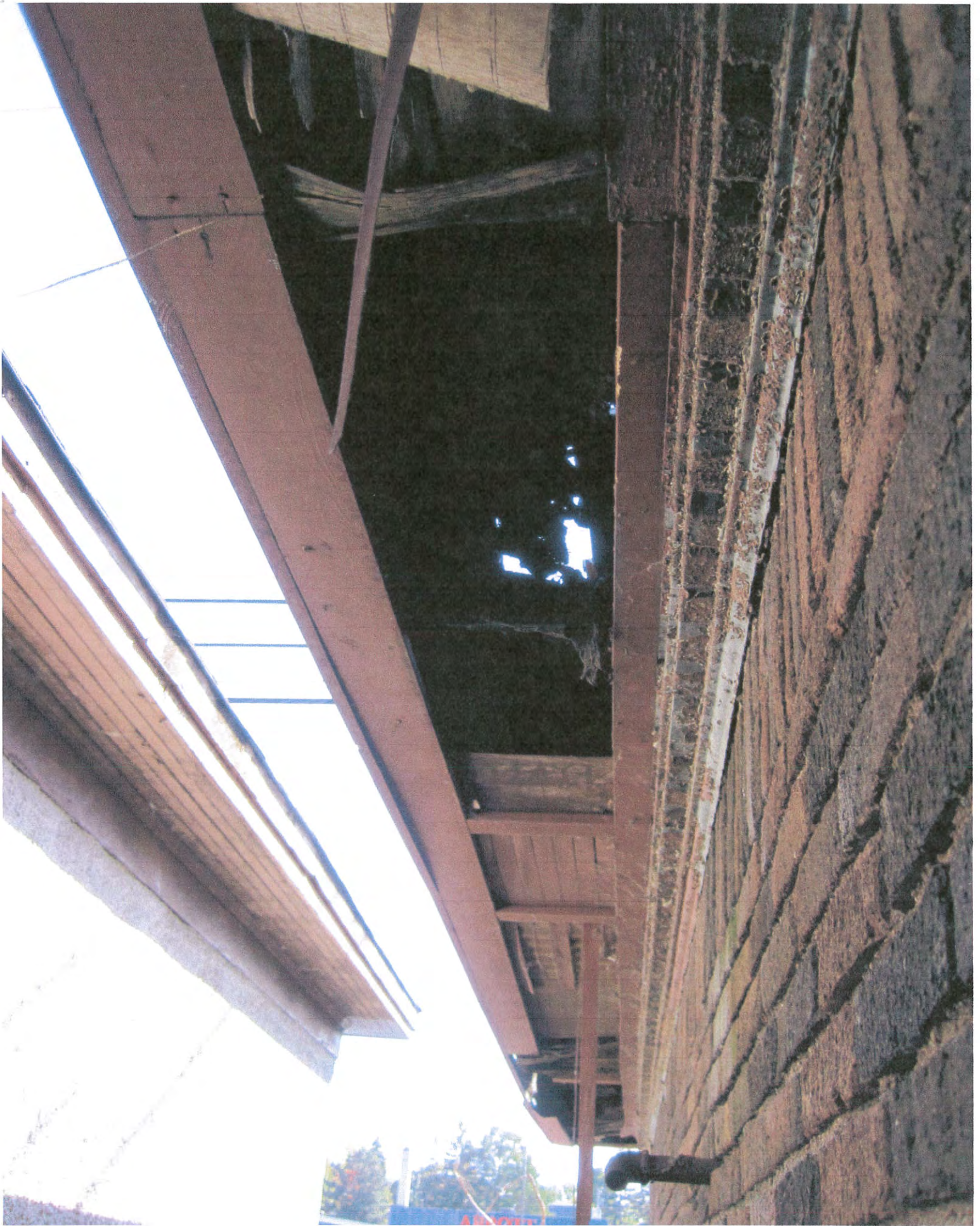
East side 50 ft. view
