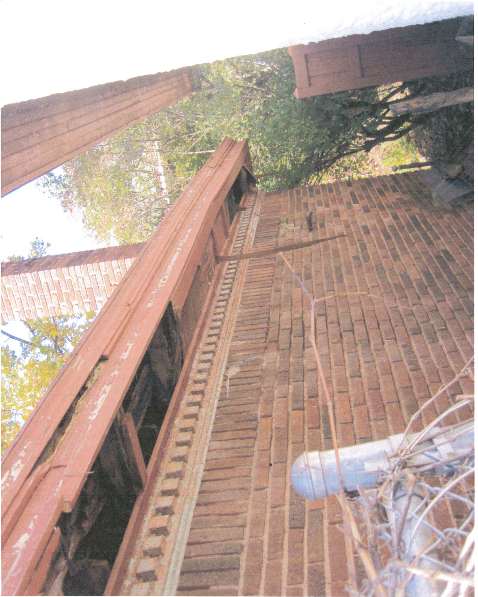
East side soffit view 2
