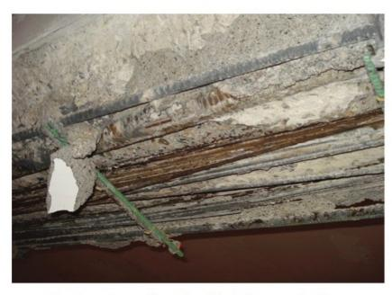
Due to rain, salt and outdated ramp design, chlorides have penetrated the concrete, causing the supporting steel to rust and the concrete to corrode and flake or break off. Photo taken as the beam was in the process of being repaired.
