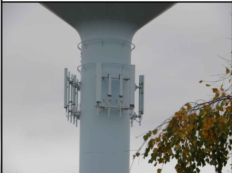
EXISTING OTHER CARRIER PANEL ANTENNAS
