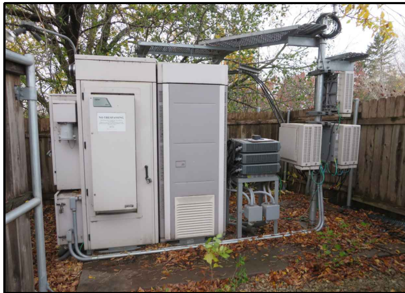
EXISTING T-MOBILE EQUIPMENT
