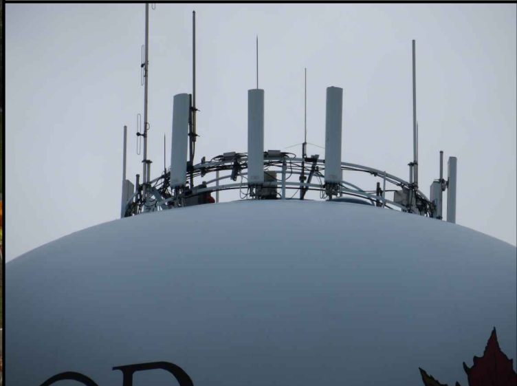
EXISTING T-MOBILE PANEL ANTENNAS @ 114'-0"
