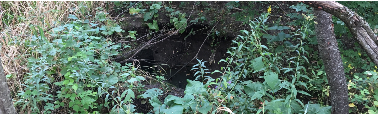
Sinkhole along Centerville 54-inch concrete conduit alignment
