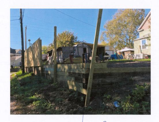
Fence that has been replaced. Shows green treated lumber and shoring posts. This material is planned to replace current gate. Current gate has been secured with lock and bar on inside of fence.
