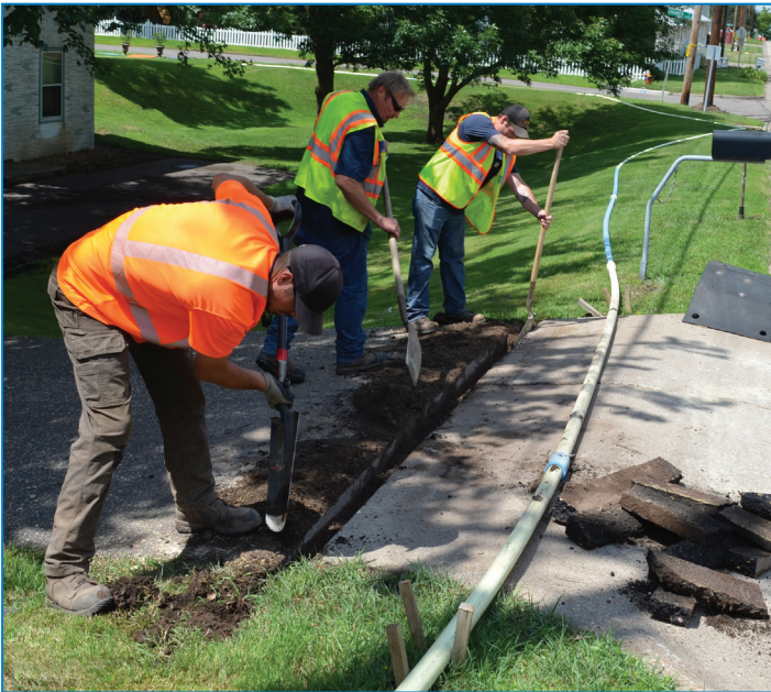
From left, Greg Sorenson, water system worker, and Pete Trooien and Travis Seidl, water utility workers, dig a trench to lay temporary water main in a driveway to allow cars to drive over it. The work was done along Larpenteur Ave. near English Street on June 30.
