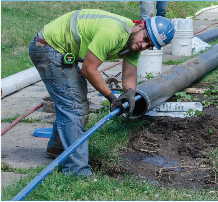
Alex Zinos, water utility worker, swabs out the water main with a chlorine solution prior to laying it at Atlantic Street near Idaho on June 30. Dustin Schluessler, water system worker, was the foreman on the job site with Sean Diesterhaft, water system worker, and Matt Schmidt, water utility worker, laying the main.
