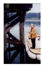
Structural assessment and rehabilitation efforts require close examination of existing wood foundation piles. We have investigated pile condition in terrestrial, fresh water, and marine environments.
