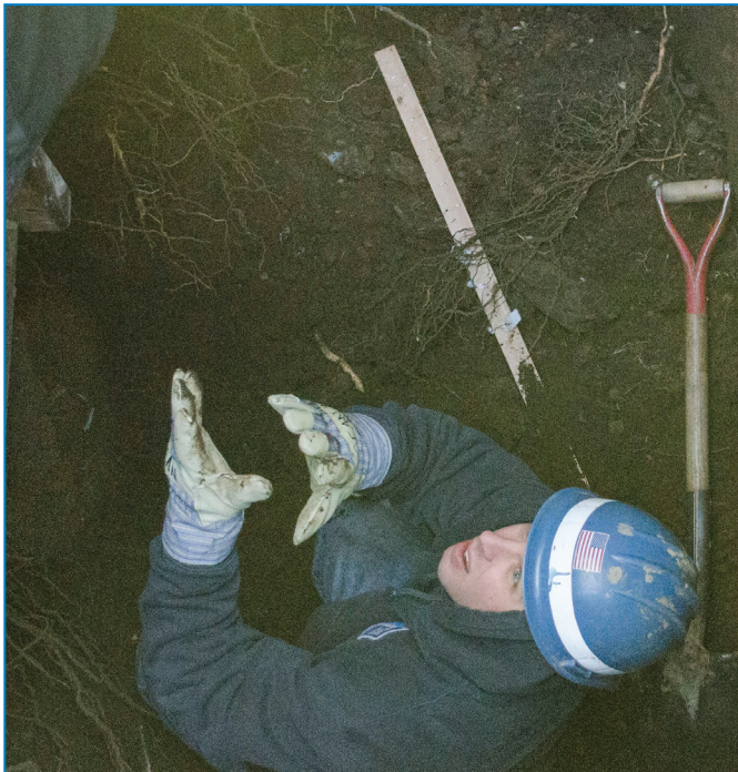
Sean Diesterhaft, water system worker, waits to catch tools that are being dropped down to him as he works inside a safety box at 800 Iglehart where Tony Palumbo's crew was replacing a shut-off valve on Feb. 15.
