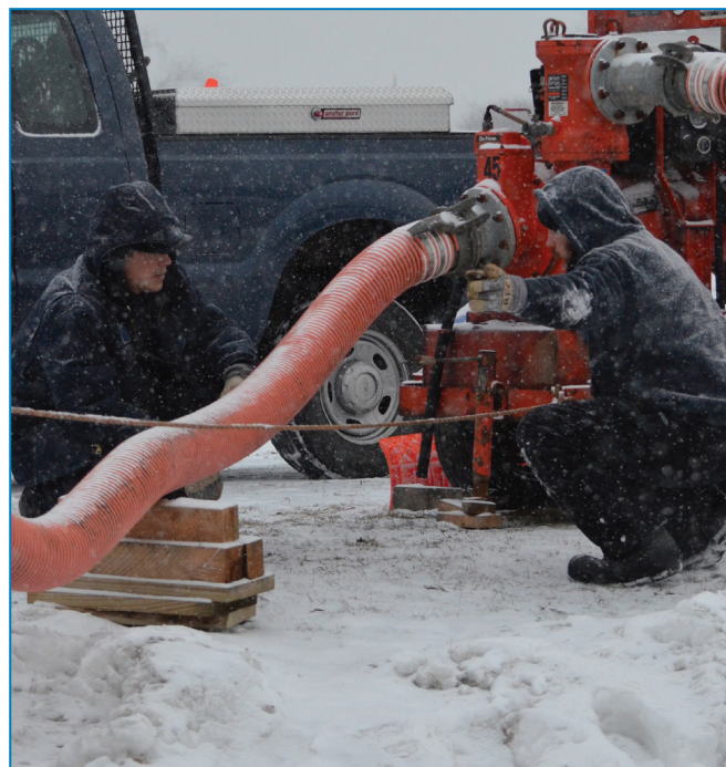
Kevin Romero and Jon Beck, water utility workers, pump water from the north finished water reservoir at McCarrons. The reservoir is being emptied in order for work to be done inside, including cleaning, and moving the chemical feed point and sampling point location. The reservoir was last open about 10 years ago in conjunction with the installation of the granulated activated carbon filters.
