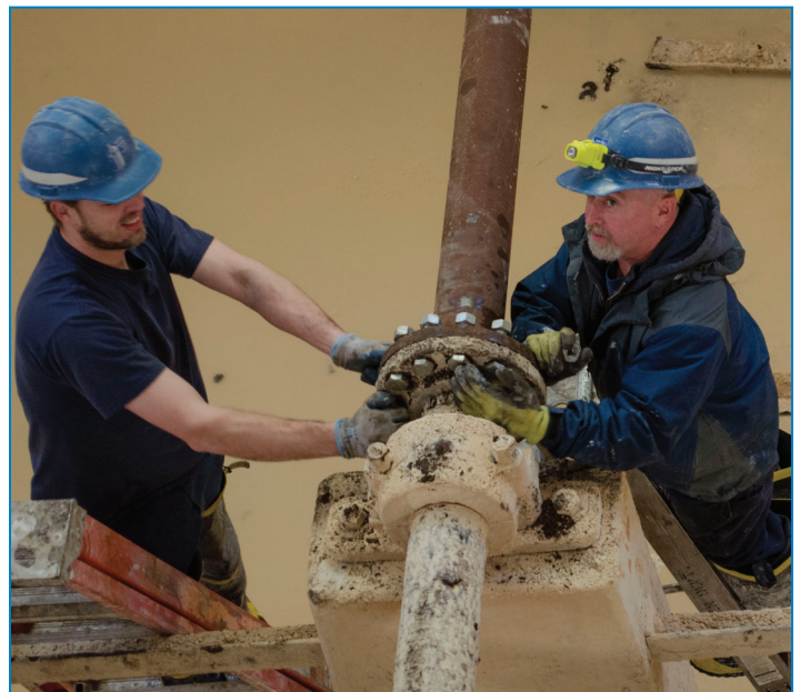
Jon Henrickson, left, maintenance worker, and Rob Ralston, water utility worker, screw bolts into the flanged pipe shaft in floc three on Dec. 28. The shaft sheared off and was replaced. The work is part of the annual maintenance that plant workers do during the slower winter months. Ralston typically works in distribution, but transferred to the plant for the winter to assist with the maintenance. Ralston has been working in the plant since Nov. 28.
