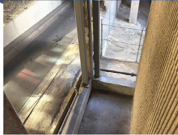
Shored up concrete NE support column with steel post
