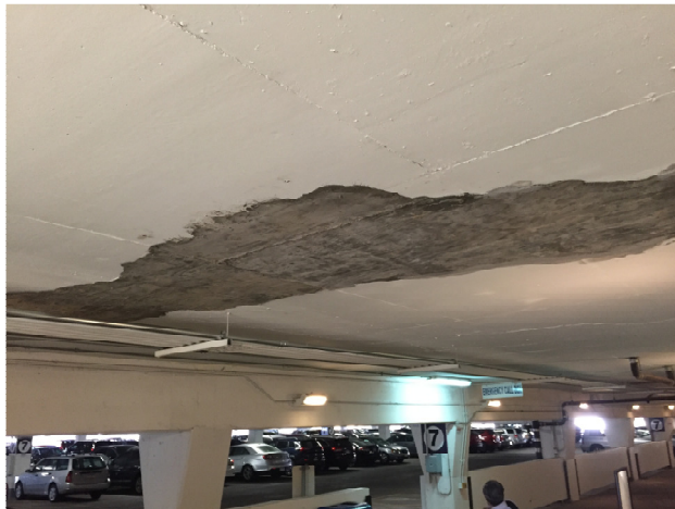
Repair overhead concrete at ped ramp
