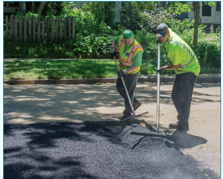
Mark Coulter and Erik Sorenson, water utility workers, spread hot asphalt to patch a hole in the street after a partial lead service line replacement in June. Rich Reeves was the truck driver.
